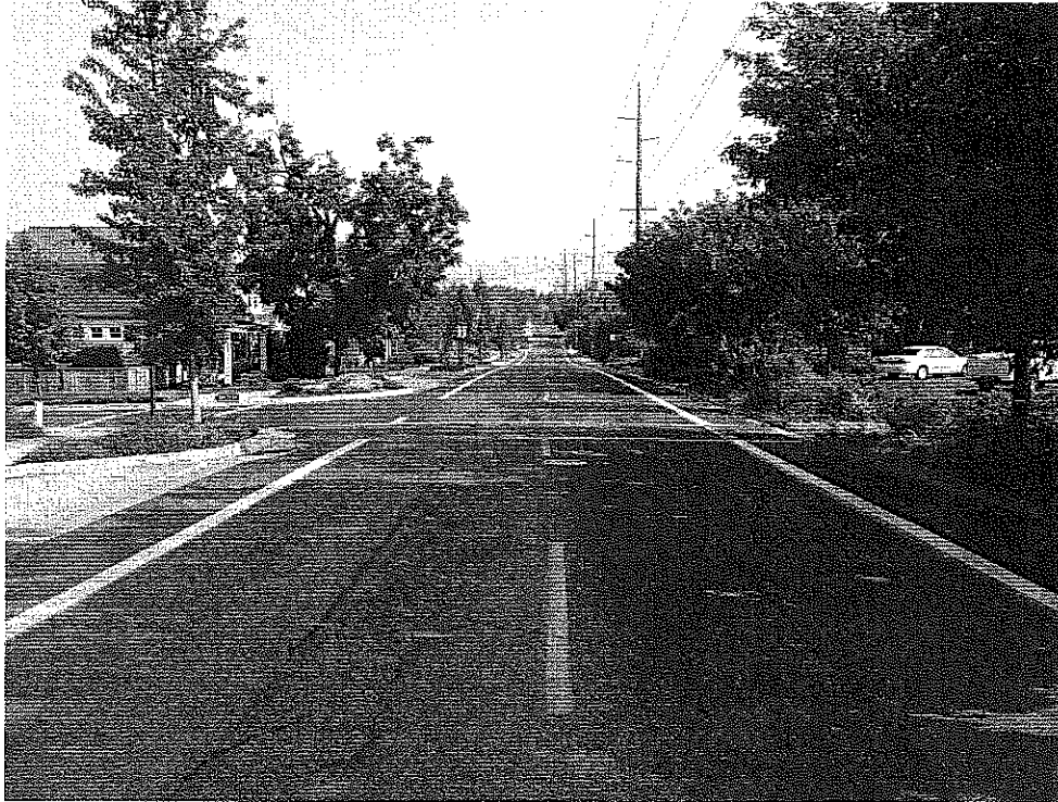
Crosswalk at Briscoe looking north
