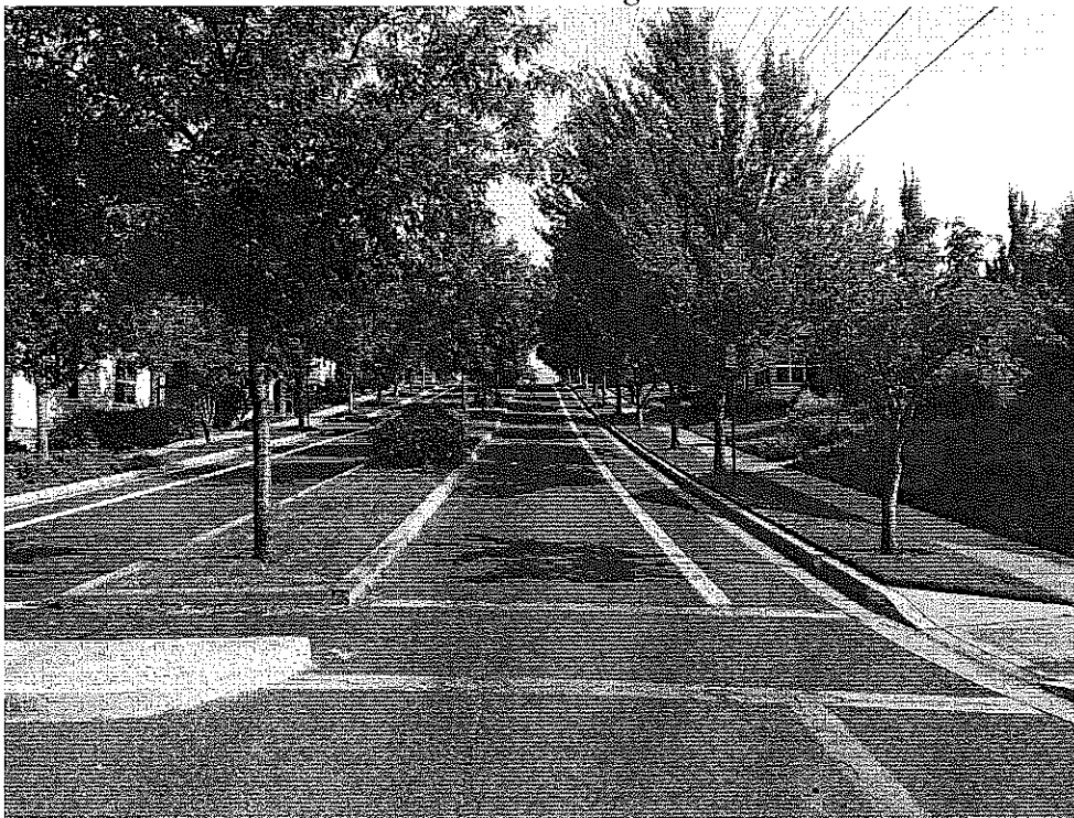
Corridor view at Mountain Meadows looking north
