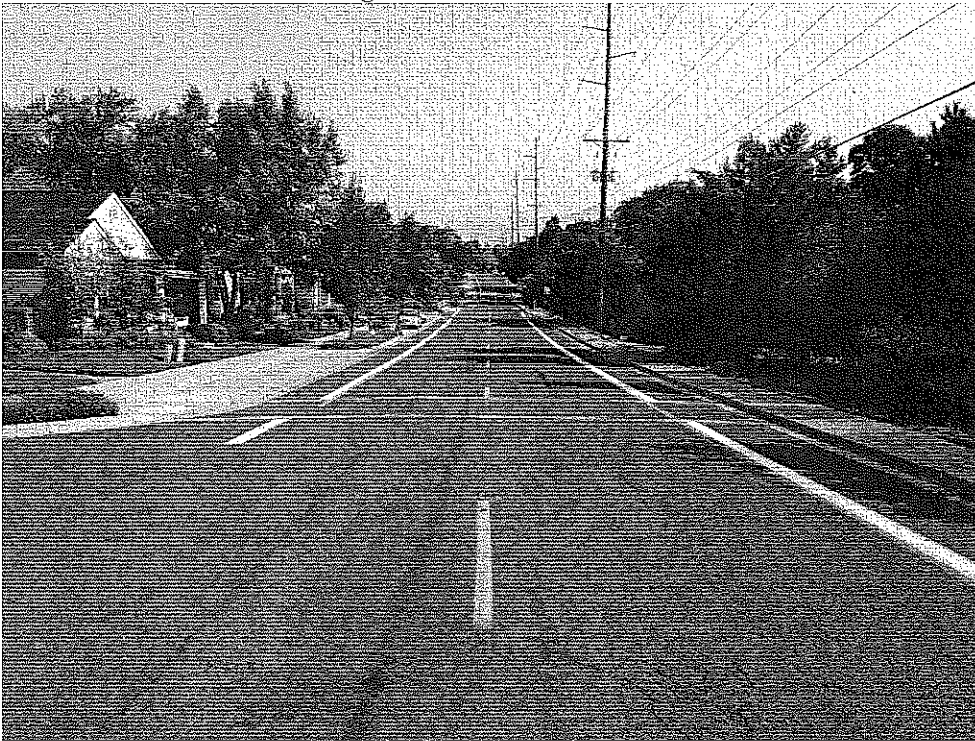
Crosswalk at Clinton looking north
