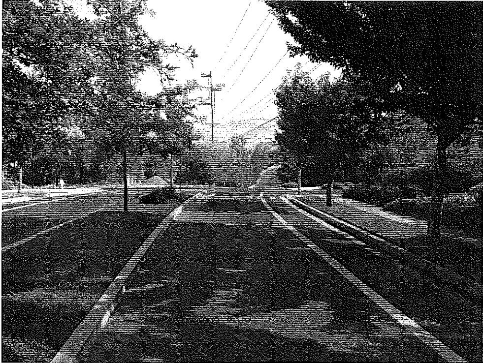
Crosswalk at Fair Oaks looking north
