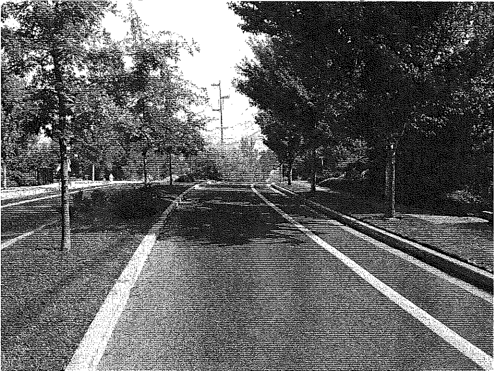
Corridor view looking north towards Fair Oaks crossing
