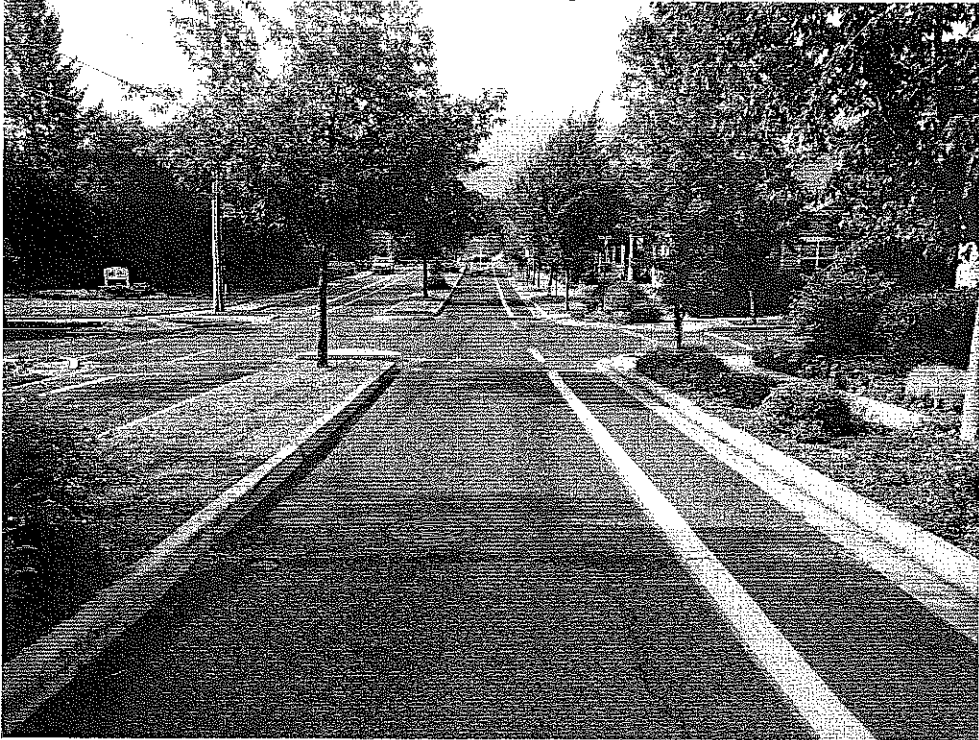
Corridor view at Mountain Meadows looking south (crosswalks)
