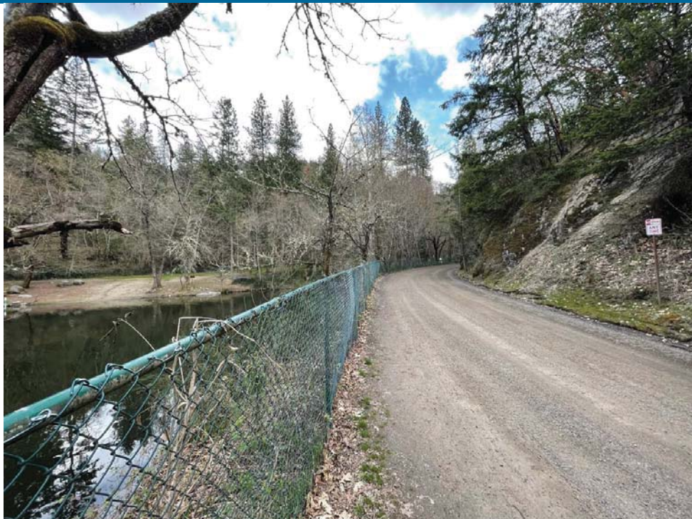
East Property Frontage on Granite Street at “Swimming Hole”
