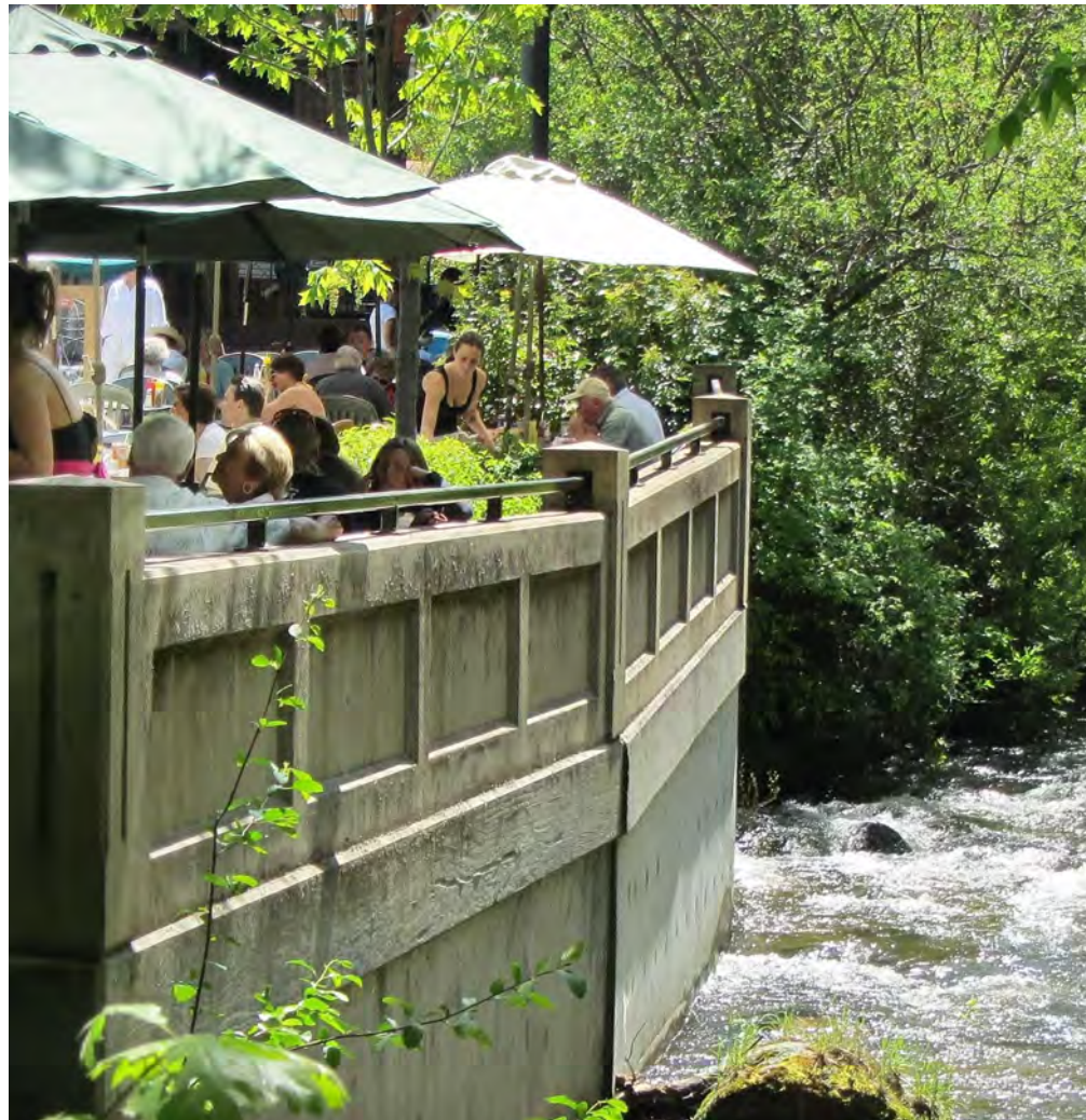
CALLE GUANAJUATO AND UPLAND DEVELOPMENT SEPARATED FROM ASHLAND CREEK BY WALLS
