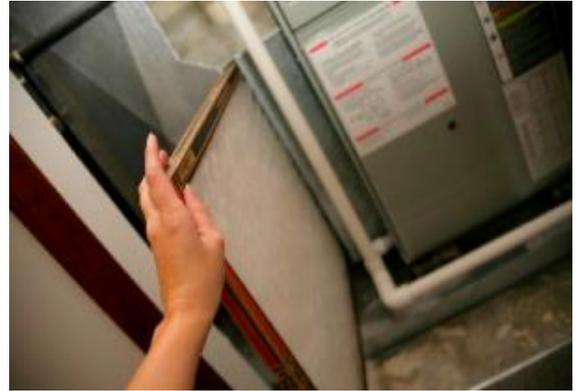
Most air conditioners are designed by default to re-circulate indoor air. **Systems that have settings for both "outdoor air" and "re-circulate" need to be set on "re-circulate" during wildfire and smoke events.**
