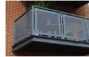
7 PERFORATED METAL RAILING MATERIAL PRECEDENT
