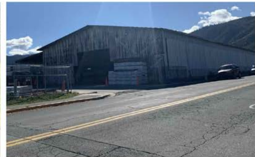
3 Ashland Lumber SCALE: LARGE MATERIAL: VERTICAL WOOD, GABLE ROOF USE: COMMERCIAL
