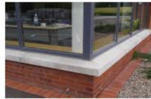
10 PRECAST CONCRETE SILL MATERIAL PRECEDENT
