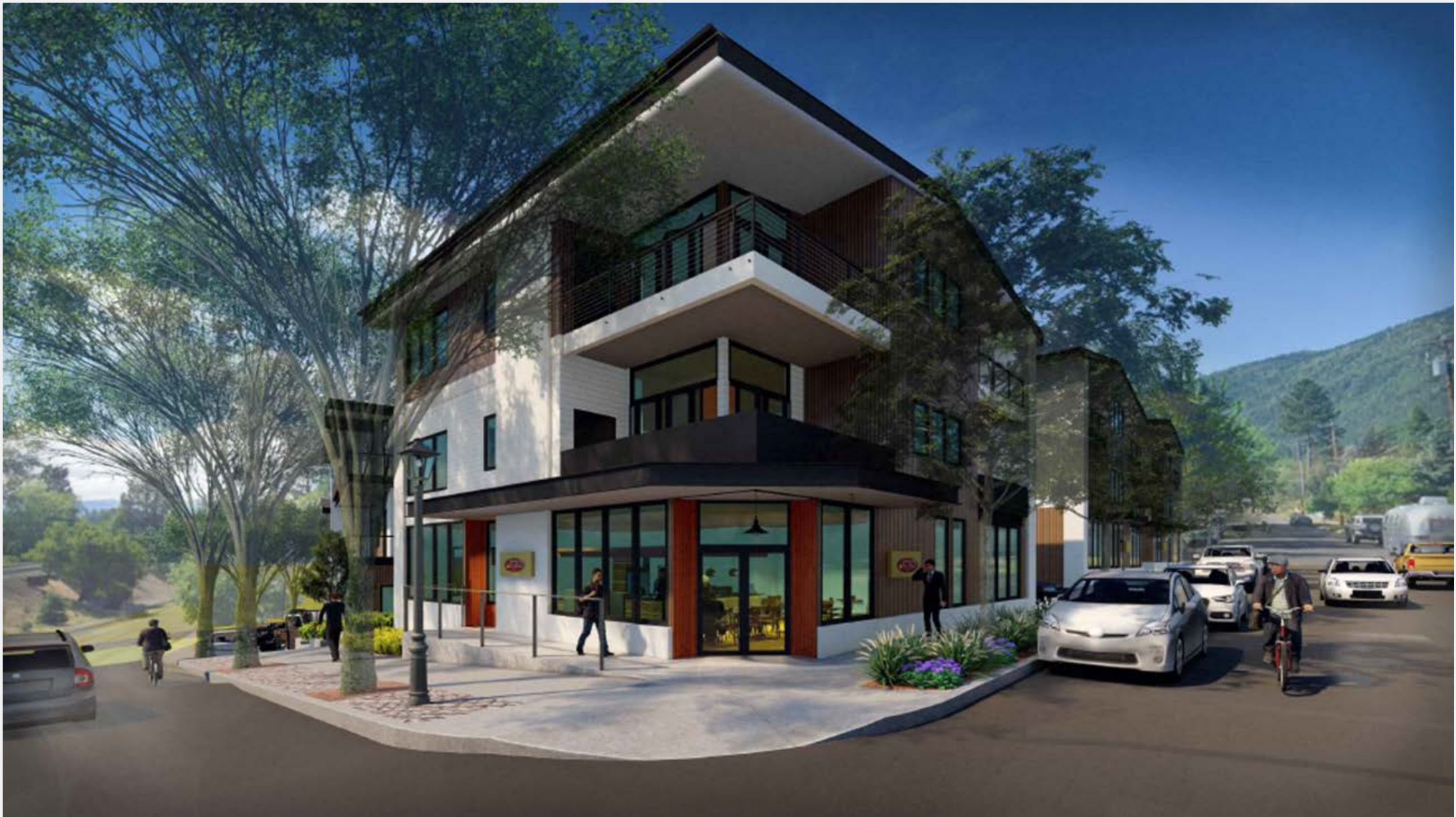
BUILDING I – HELMAN STREET AND VAN NESS INTERSECTION
