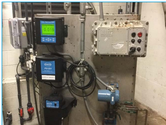
Photo 3-24 – Dual Media Filter #1 Turbidity Meter
