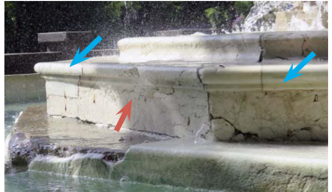
Crack (red) and dutchman repairs (blue) in lower bowl. Note the open joint between the plaster and the marble.
