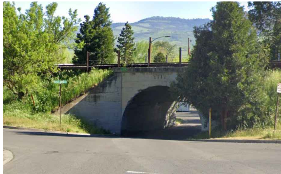
2 Tunnel Under Rail SCALE: MEDIUM MATERIAL: CONCRETE, STEEL USE: INDUSTRIAL
