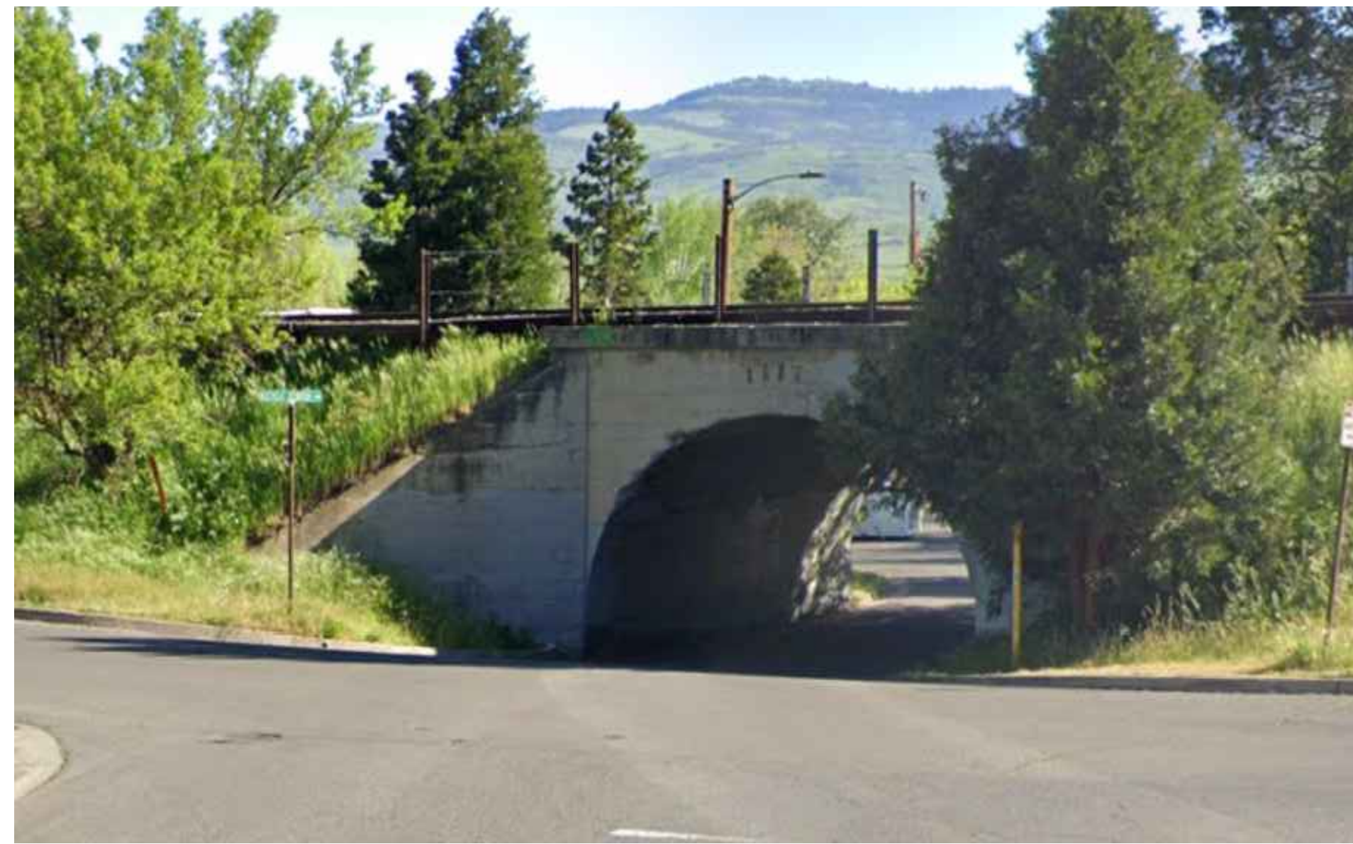
2 Tunnel Under Rail SCALE: MEDIUM MATERIAL: CONCRETE, STEEL USE: INDUSTRIAL
