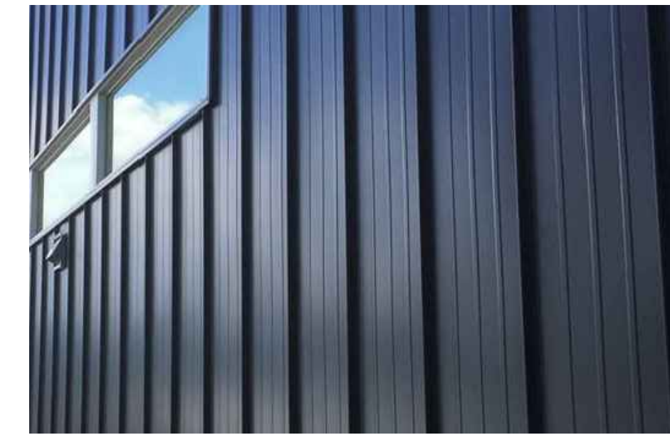
4 VERTICAL SIDING MATERIAL PRECEDENT
