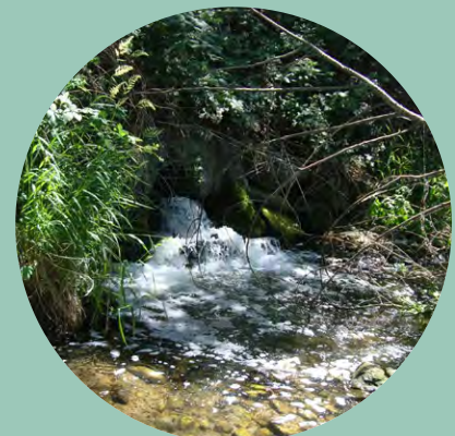
Existing outfall into Ashland Creek
