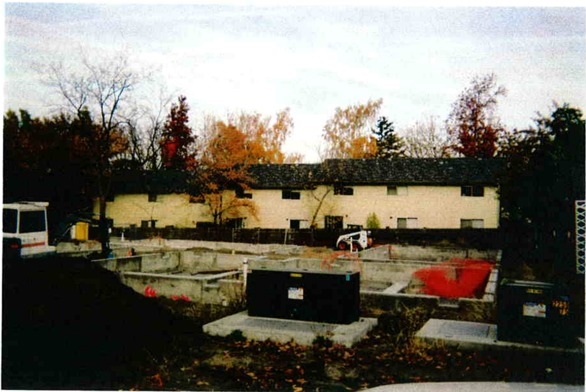
VIEW OF BACK OF UNITS FROM LINCOLN STREET
