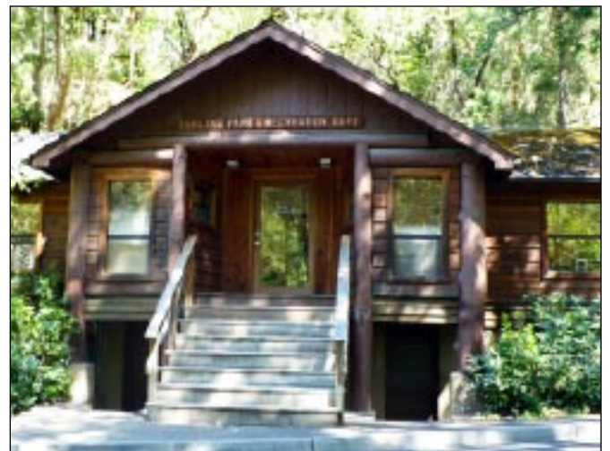
Ashland Parks & Recreation Office in Lithia Park, 340 S Pioneer St, Ashland
