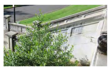
Cracks in the outer face of the staircase. This crack is also visible at the interior face.
