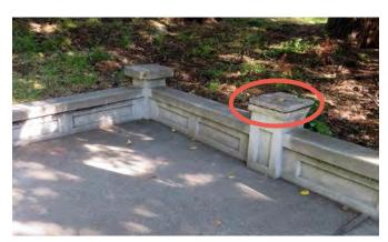
Concrete cracking, spalls, and soiling at terrace columns.
