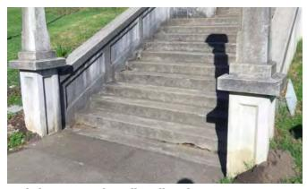
Failed repairs and small spalls at lower stairs.
