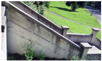
Cracks in the outer face of the staircase.
