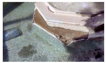
Plaster loss at concrete base. Note plaster loss below the water, on the floor of the pool.
