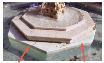
Cracks in plaster over concrete base.
