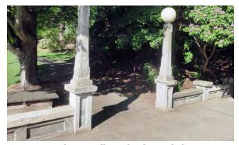
Concrete cracking, spalls, and soiling at light posts.
