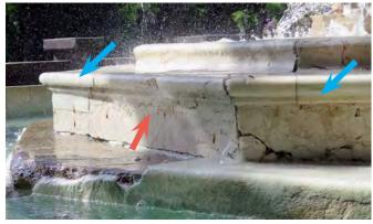
Crack (red) and dutchman repairs (blue) in lower bowl. Note the open joint between the plaster and the marble.
