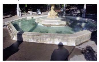
Concrete cracking, spalls, and soiling at outer rim of
