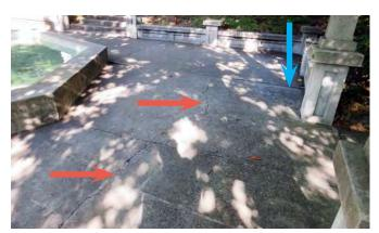
Concrete cracks (red) and warped wood strips in terrace floor (blue).
