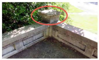
Concrete cracking, spalls, and soiling at terrace column.
