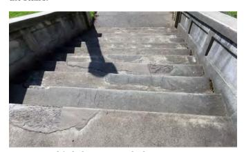
Uneven and failed repairs at the lower stairs.
