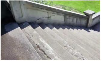
Cracks in cheek wall and failed repairs and cracks in the stairs.
