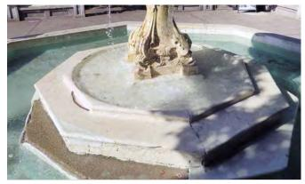
Previous repairs and open joints at lower bowl. Note the plaster failure and exposed concrete at the bottom right.
