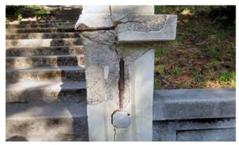
Concrete cracking and spalls at light post.
