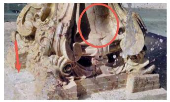
Weathered veining in lower pedestal. Note the dutchman repair indicated with an arrow.
