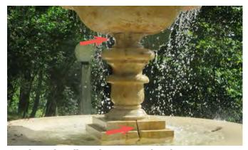
Cracks and spalls at the upper pedestal.
