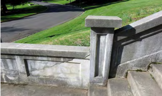
Cracks in the cheek wall. This crack is also visible at the exterior face.
