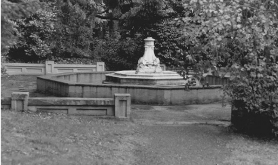
Butler-Perozzi Fountain, circa 1981 before restoration. Note the missing light posts and fountain bowls.
