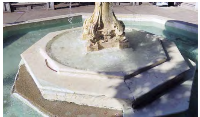
Previous repairs and open joints at lower bowl. Note the plaster failure and exposed concrete at the bottom right.
