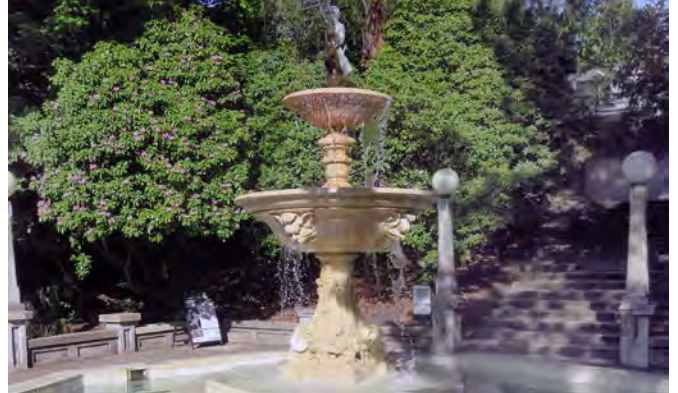
Water flows unevenly off the north east edges of the bowls. Note that the flow out of the lions is not smooth.
