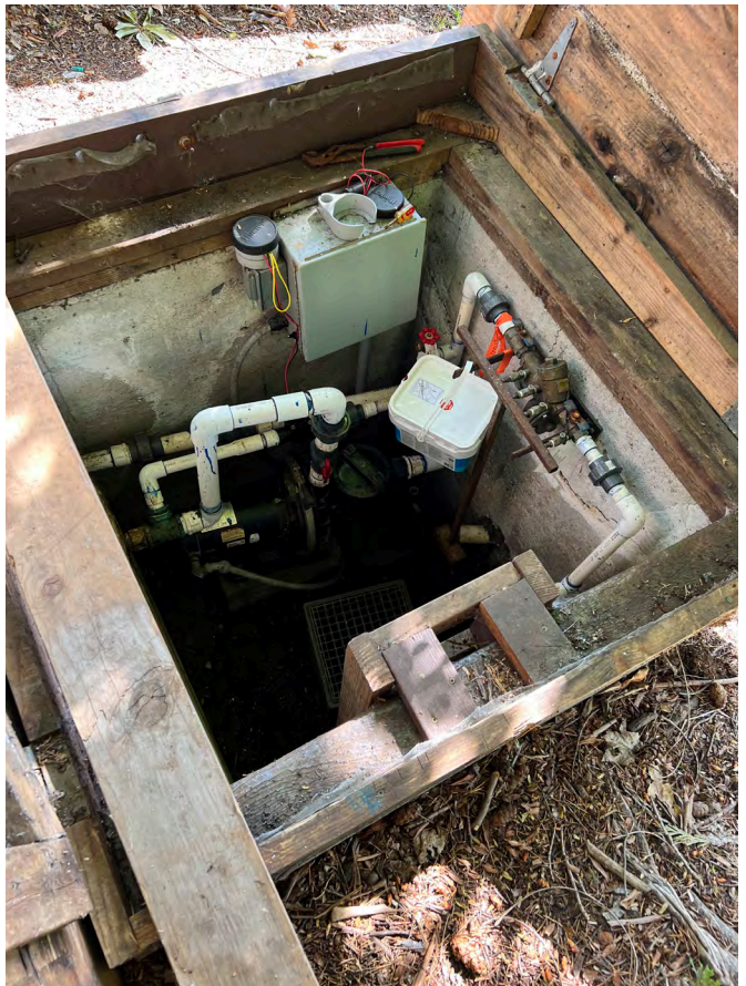
Water splashes out of the east end of the fountain, at the top of the stairs.
