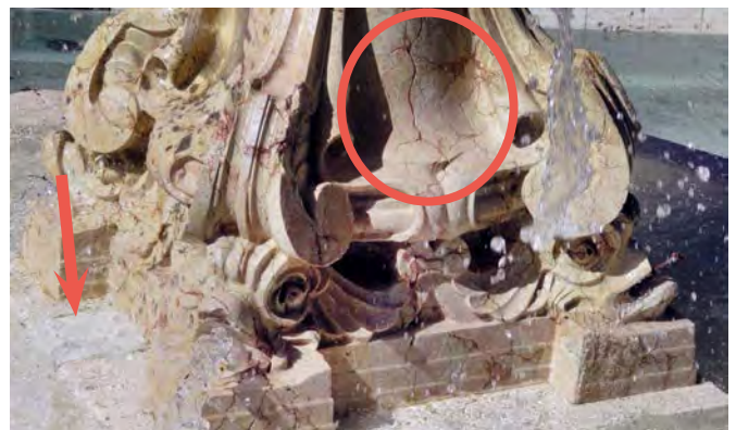
Weathered veining in lower pedestal. Note the dutchman repair indicated with an arrow.
