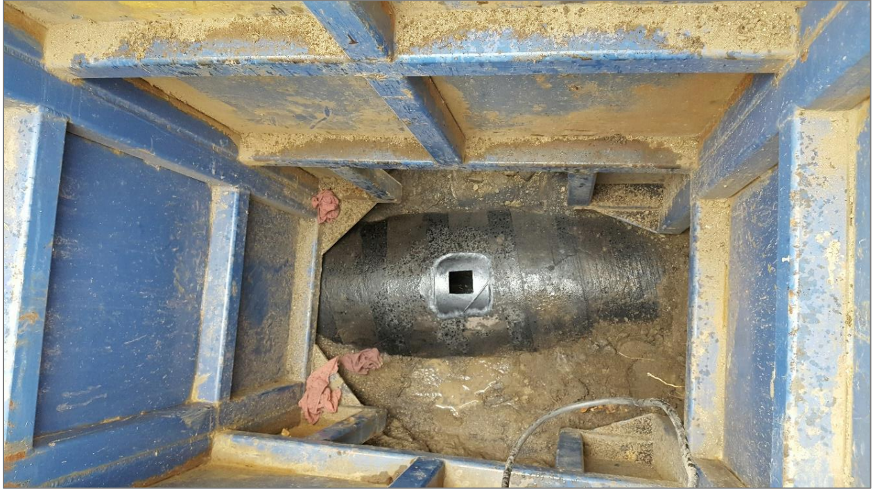
TID Pipeline Coupon Collected on Glenview Drive (Near Access Road to Concrete Pit Site)
