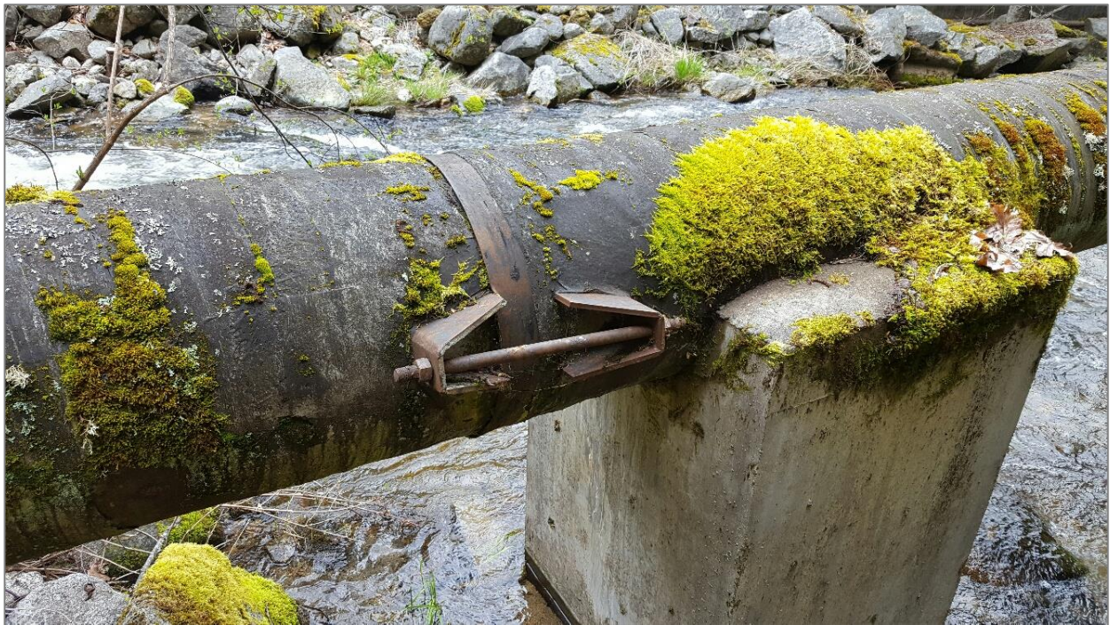
Pipe Joint Near Existing WTP
