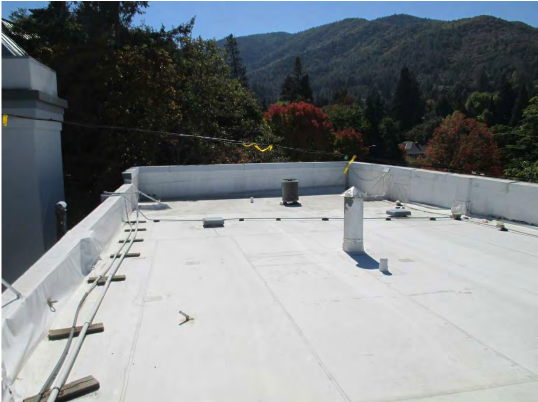
PHOTO 0217 – Main building area roof looking toward the south
