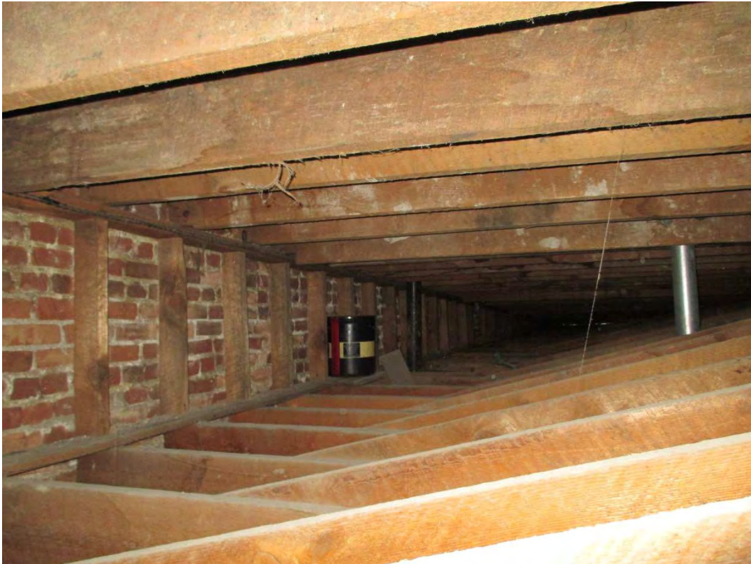
PHOTO 0264 – Main building area roof framing looking south
