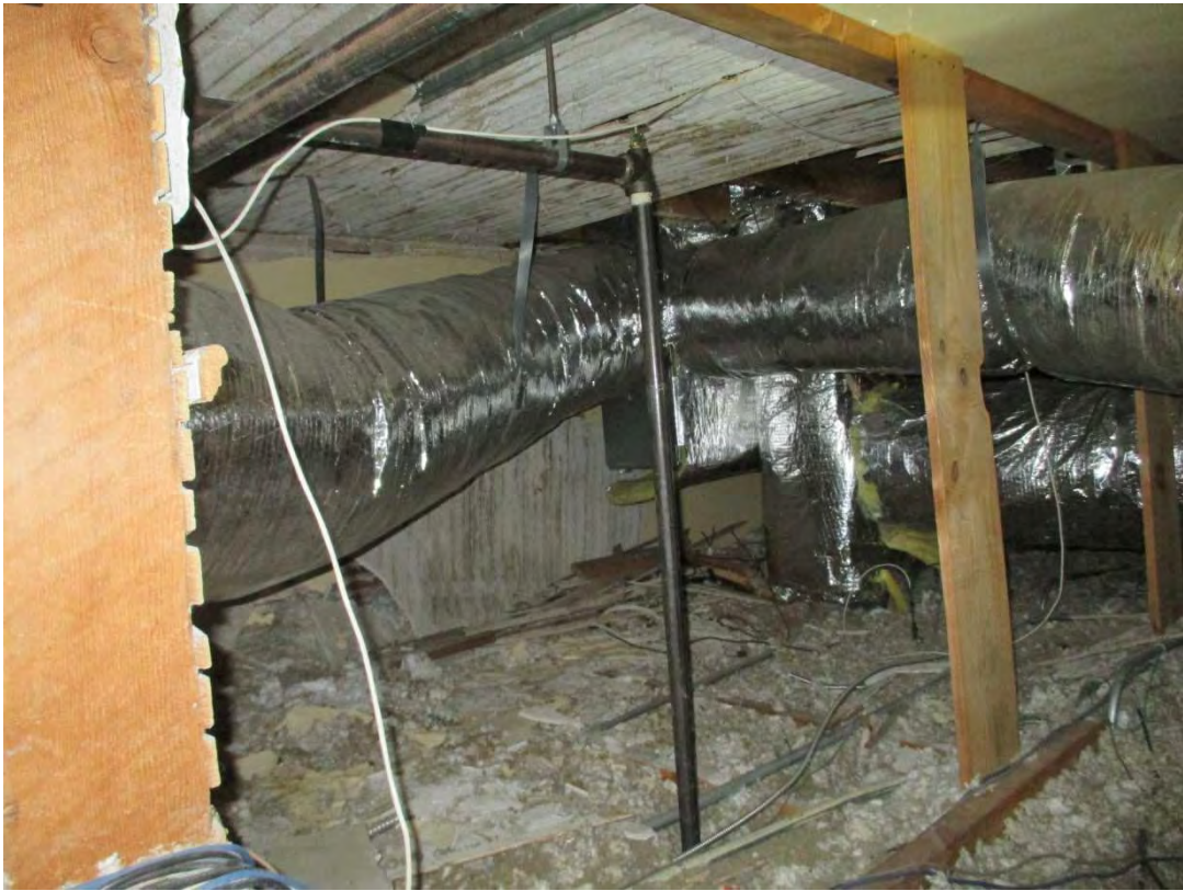
PHOTO 0263 – Upper floor ceiling cavity looking toward the southwest
