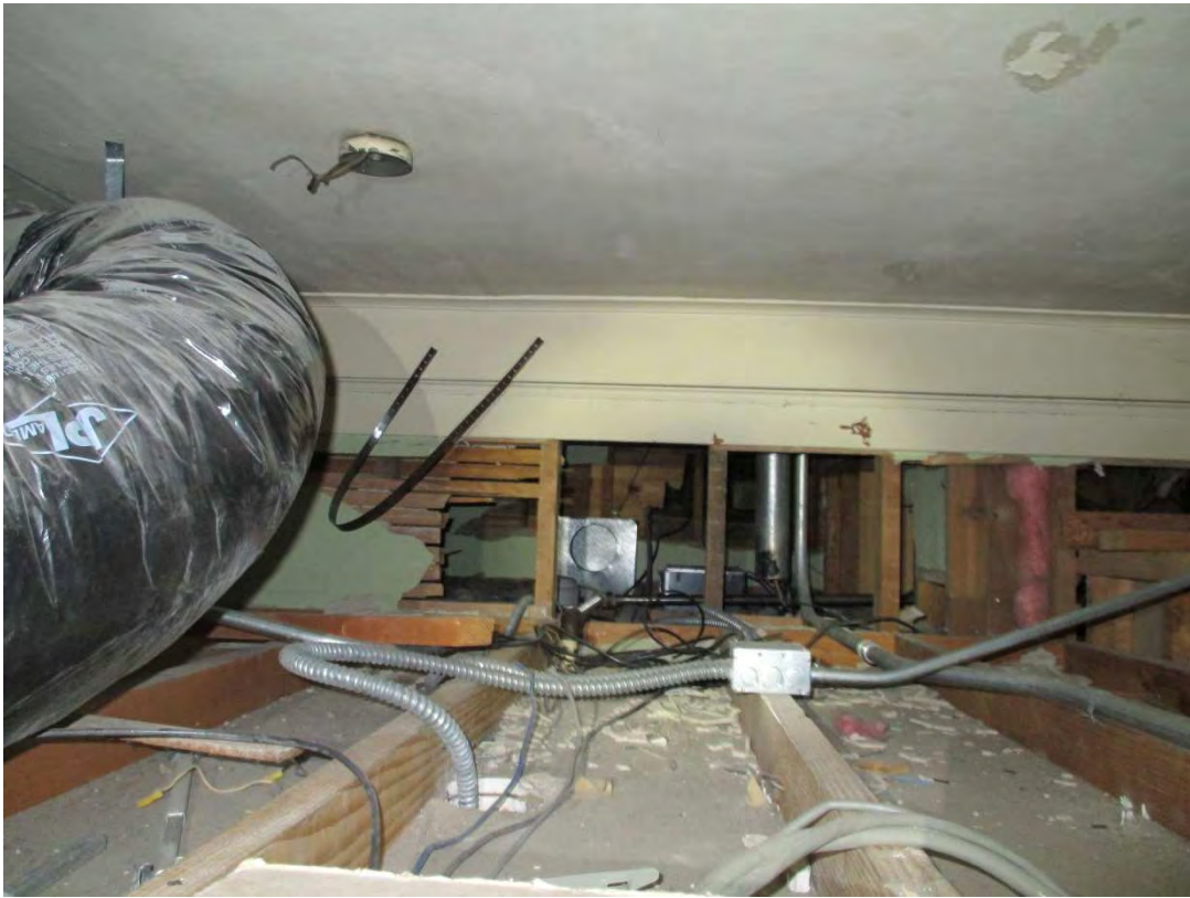
PHOTO 0244 – Main floor ceiling cavity in the main building area
