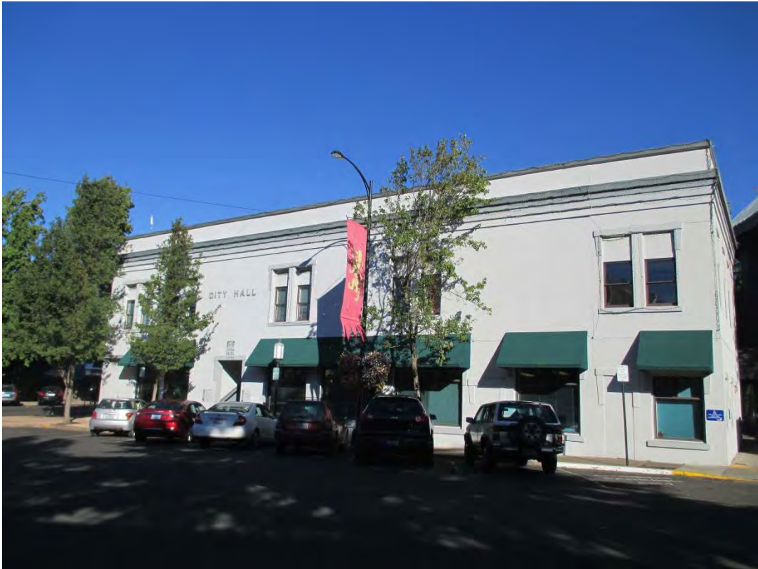
PHOTO 0291 – West elevation of the building looking toward the southwest corner
