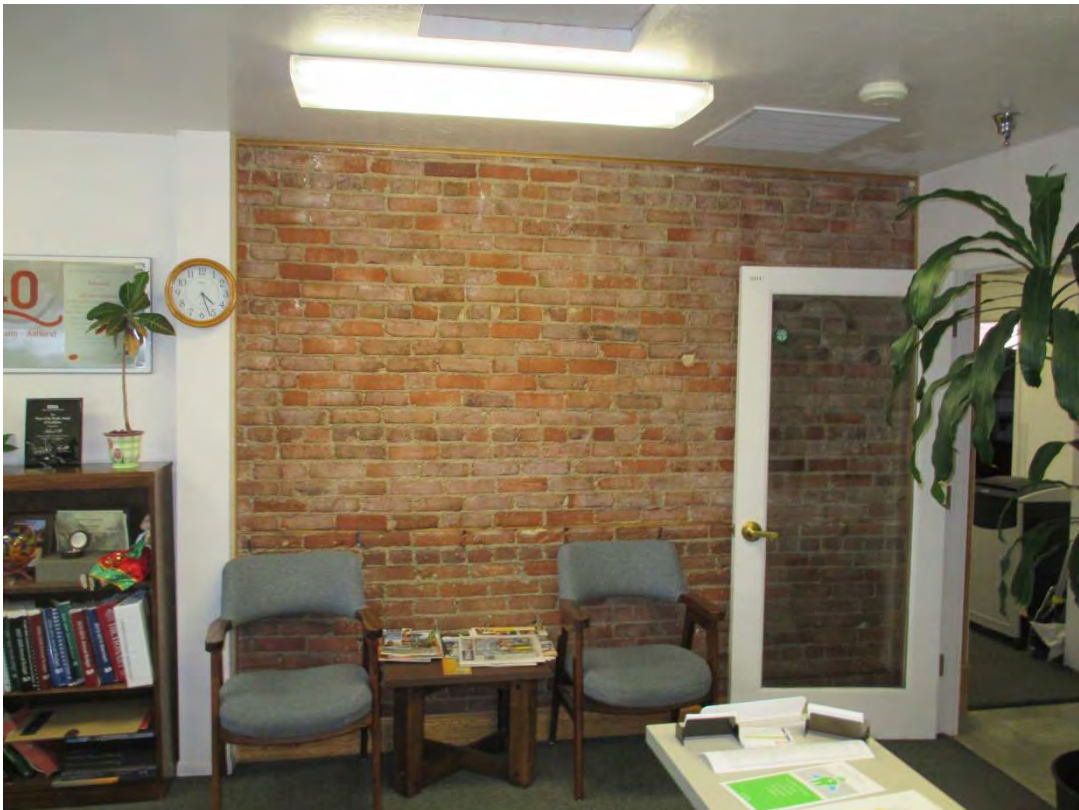
PHOTO 0285 – Exposed unreinforced masonry wall in the mayor's office vestibule
