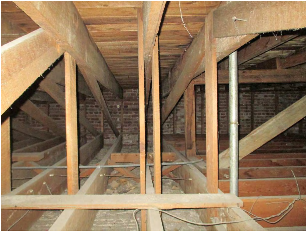
PHOTO 0256 – Main building area roof framing looking west
