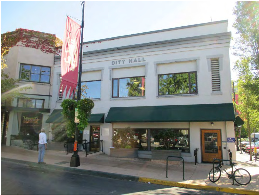
PHOTO 0234 – North elevation of the building looking toward the northwest corner
