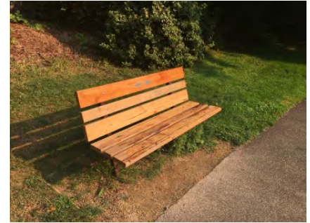
Fig.3-Embedded steel support posts w/ wood planks located in Lithia Park
