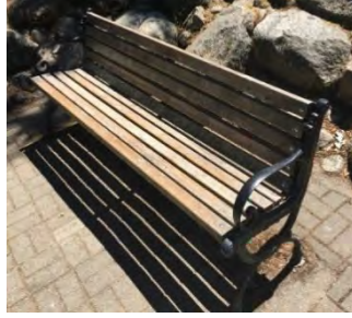
Fig.2-Partial steel frame w/ woods slats located in Lithia Park
