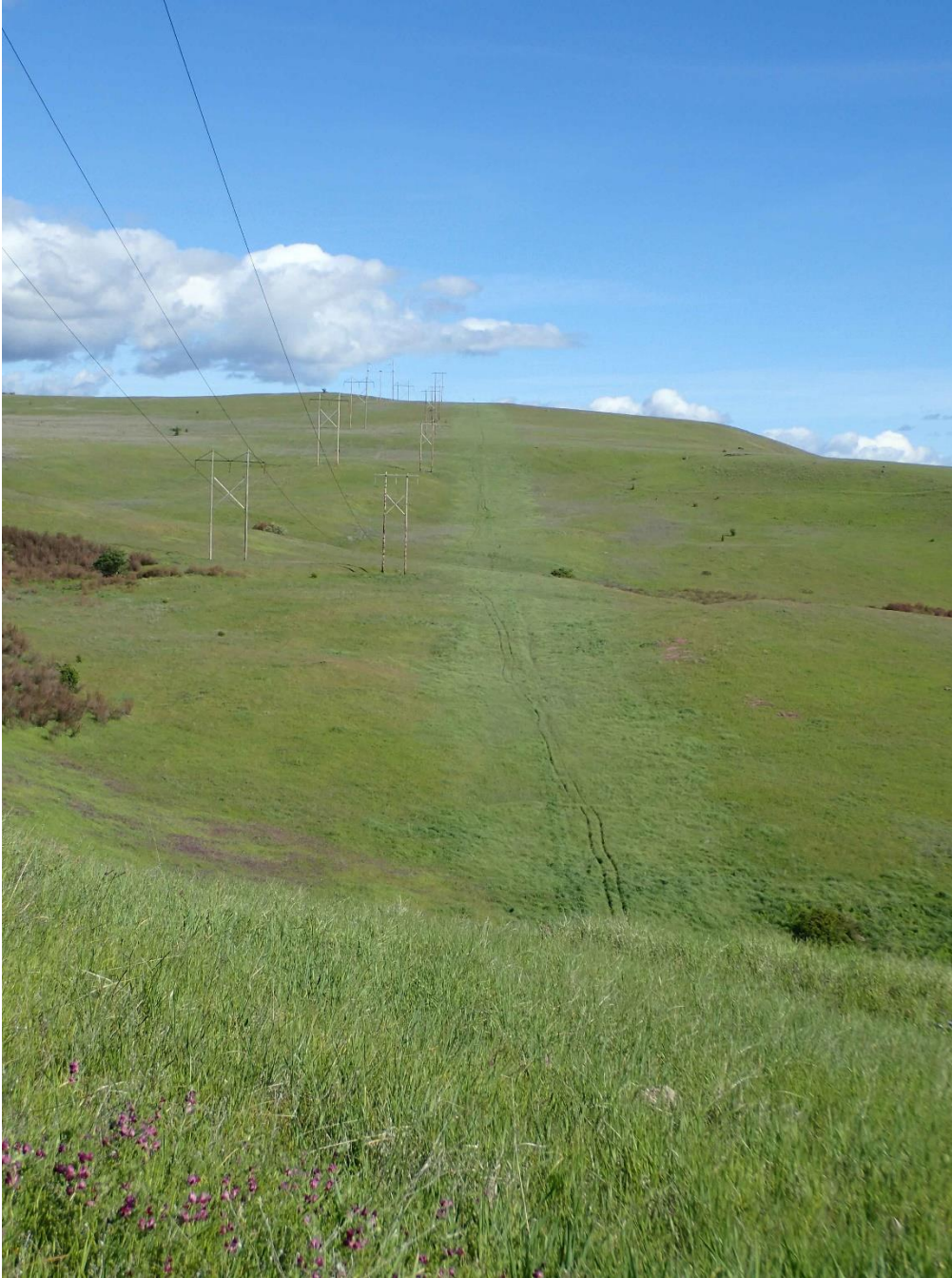
View of powerline and gas pipeline corridors on the Property; the pale strip from top to bottom, just left of center, with OHV tracks, is a Thinopyrum ponticum monoculture atop the buried gas pipeline (see 3.3 Noxious Weeds)
