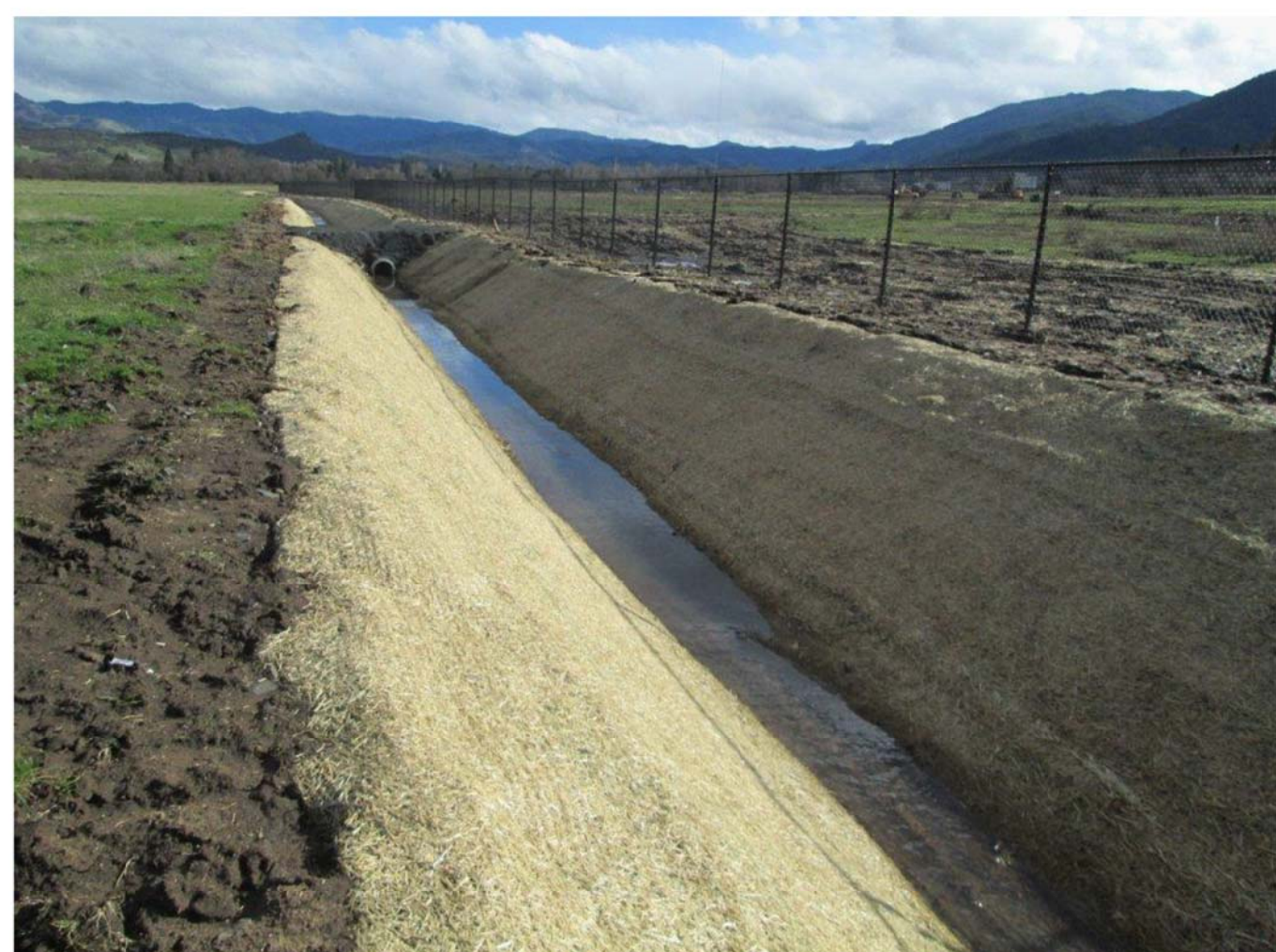
Photo B: Looking South Perimeter Irrigation Ditch & Fence
