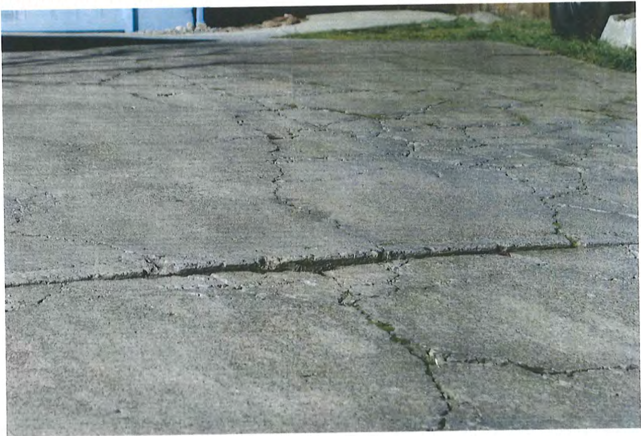
Cracking concrete driveway.
