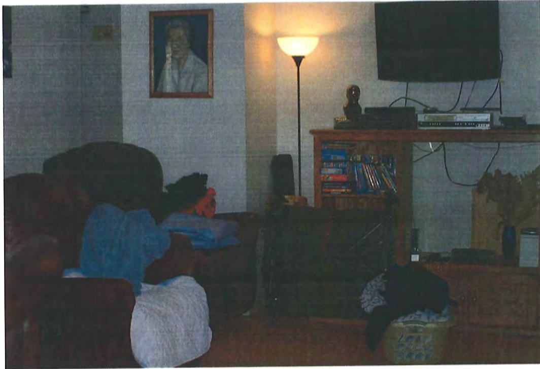
View of communal living area. Note lights on during daytime. Proposal includes the addition of skylights.
