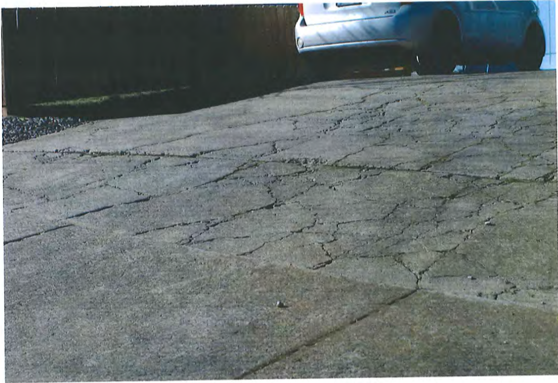
Cracking concrete driveway.
