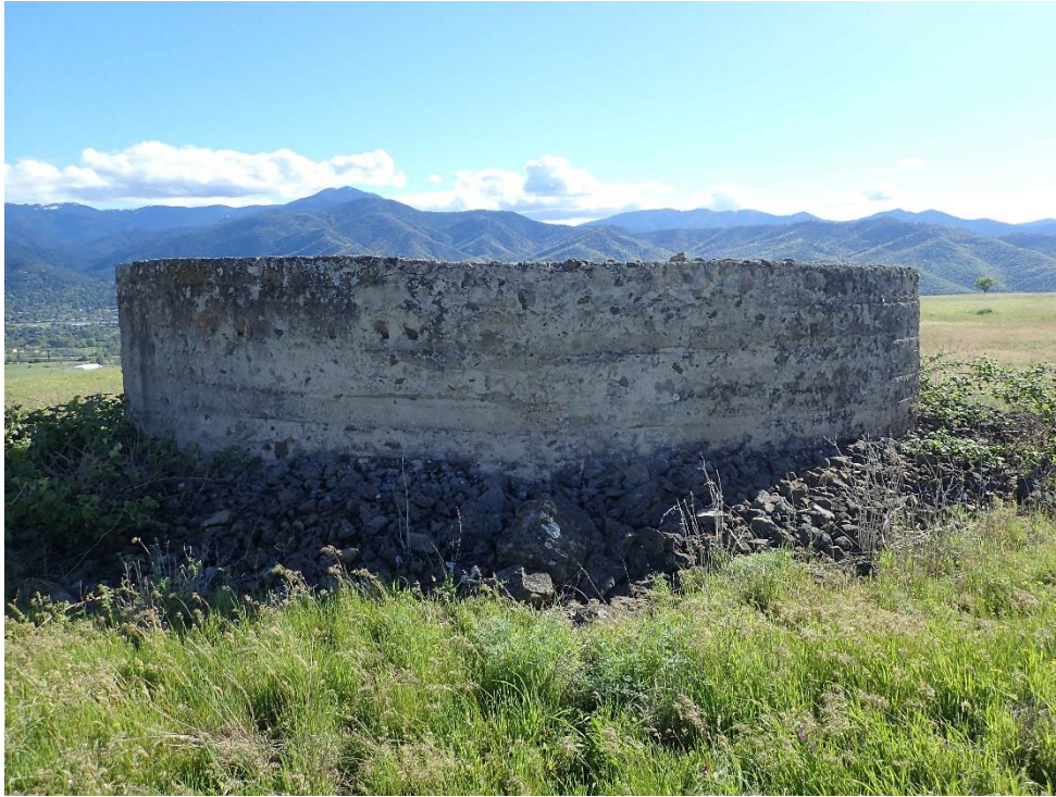
Cement “cistern” on broad ridgeline
