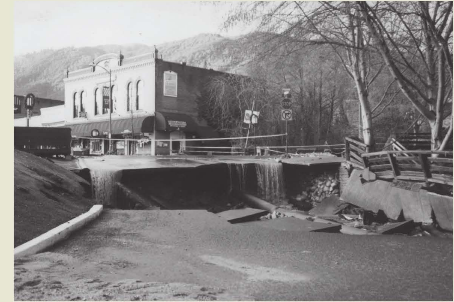
1997 Ashland Creek Flood
