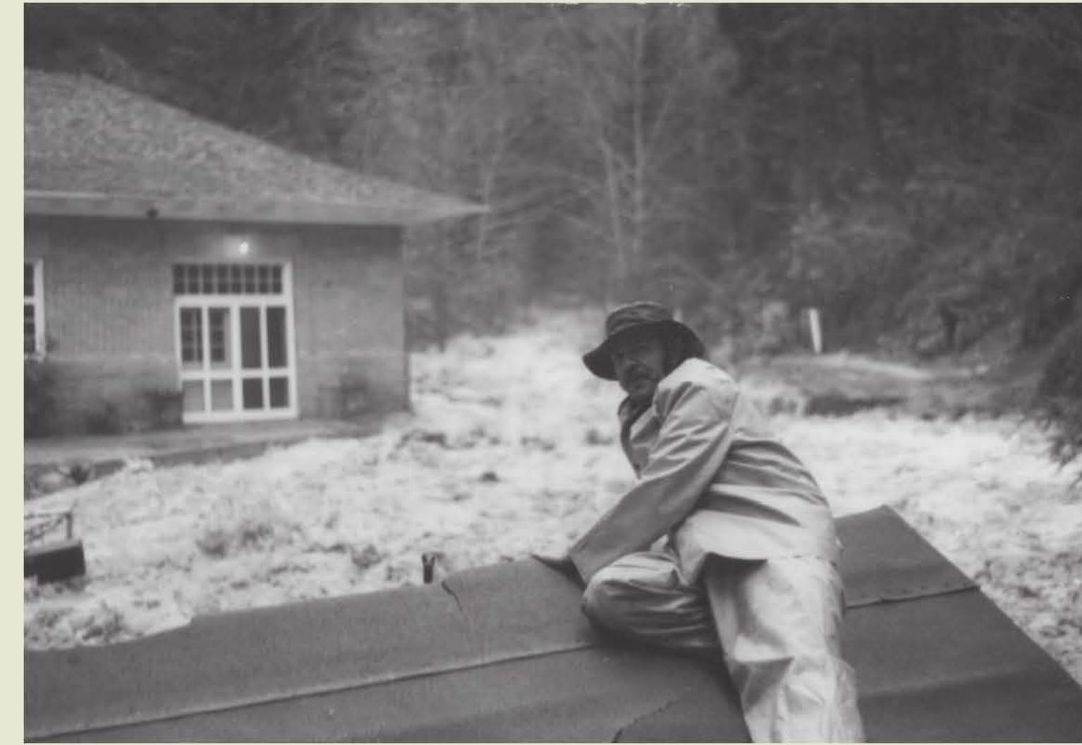
1974 Ashland Creek Flood
