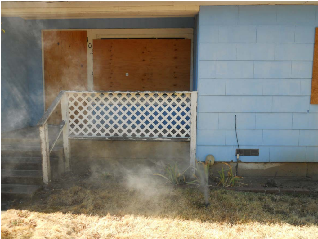
1038 Henry Street: Cleanout cap missing
