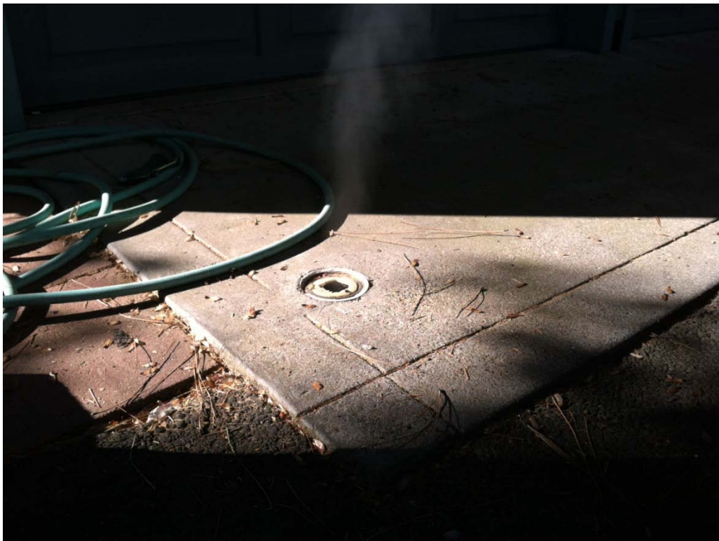
980 Morton St: Smoke emitting from broken cleanout cap
