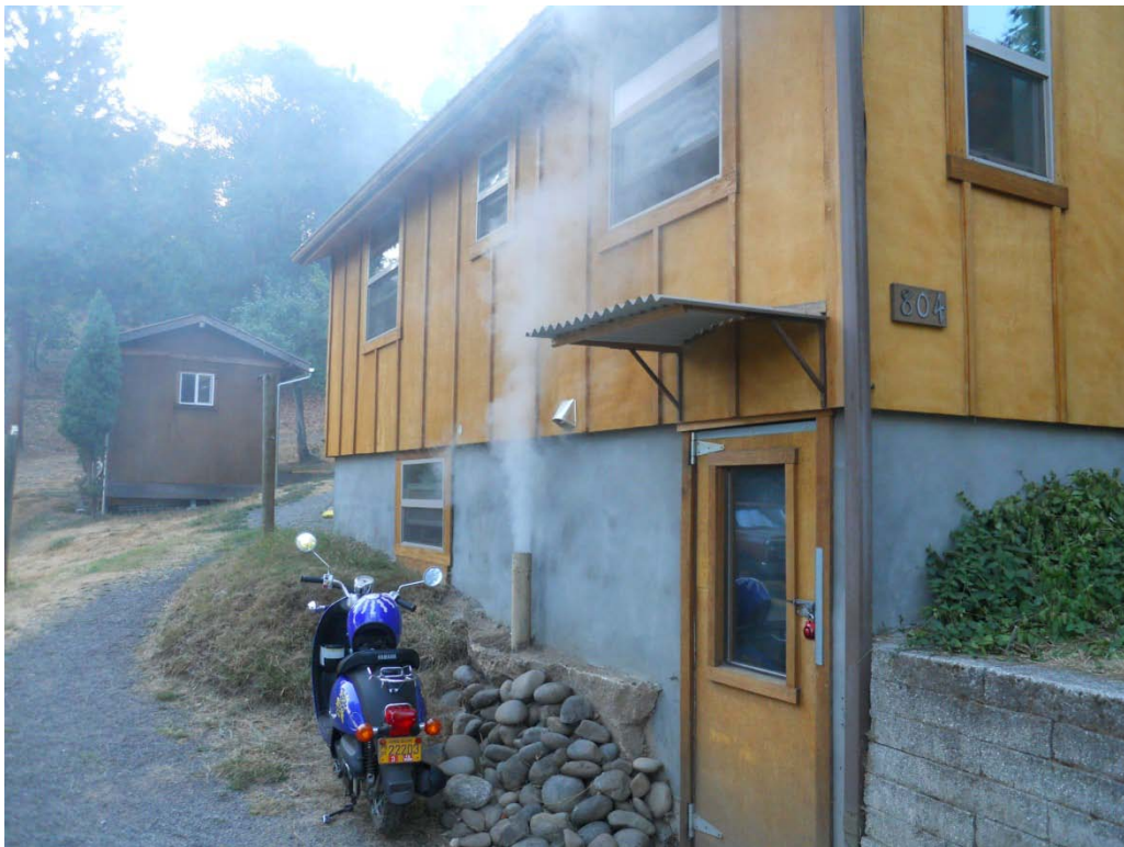
804 Beach Street: Smoke emitting from old sanitary sewer pipe lateral without cap
