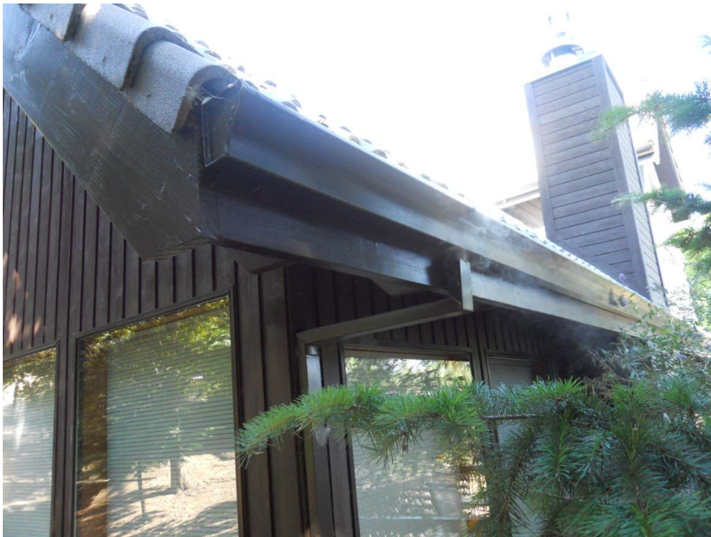
570 Weller Lane: Smoke emitting from gutters and downspouts
