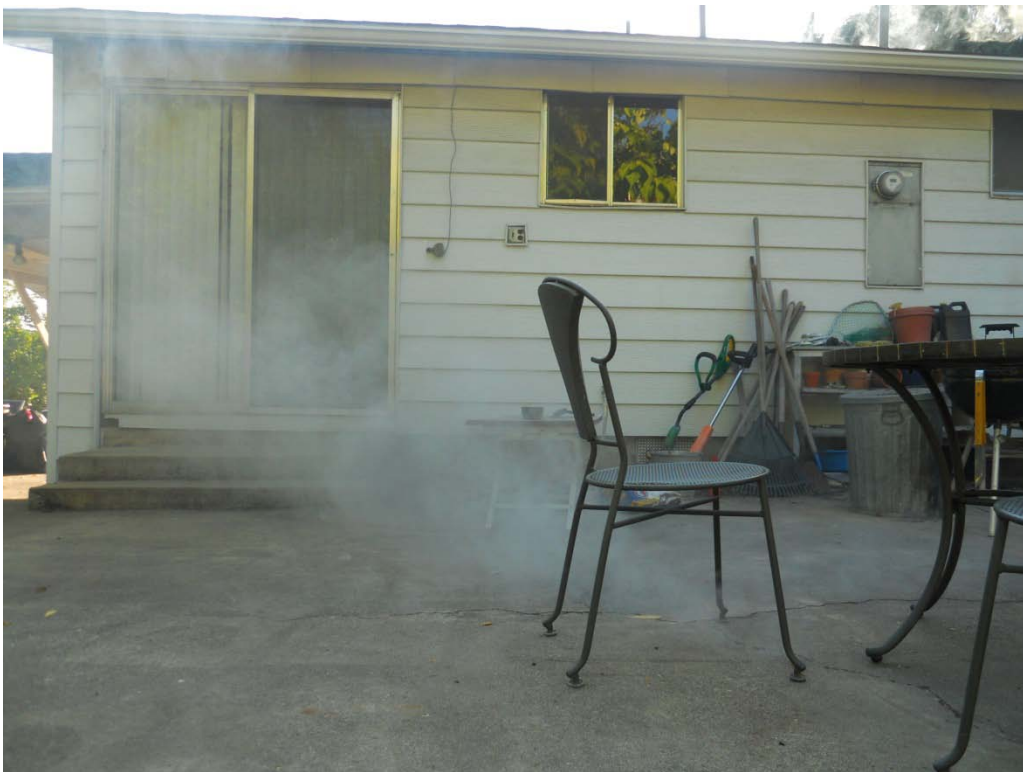
411 Euclid Avenue: Smoke emitting from crack in backyard concrete patio
