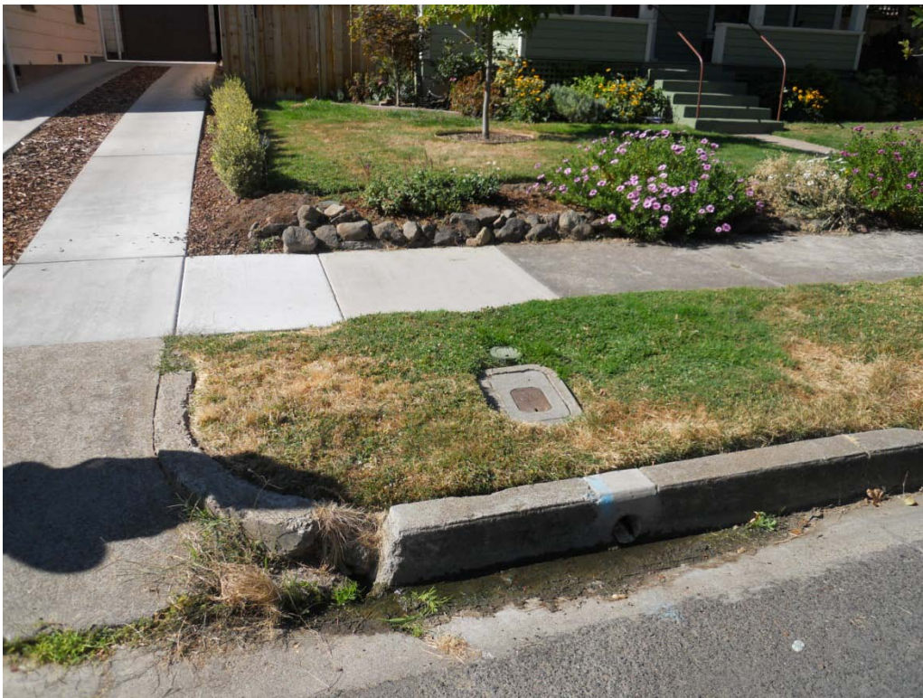
550 Allison Street: Smoke emitting from broken curb near abandoned sewer lateral
