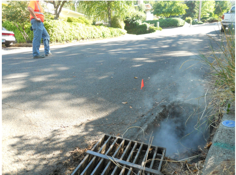
Smoke testing from this stormwater catch basin near 645 Glenwood Drive revealed a cross connection to the City's sanitary sewer system.
