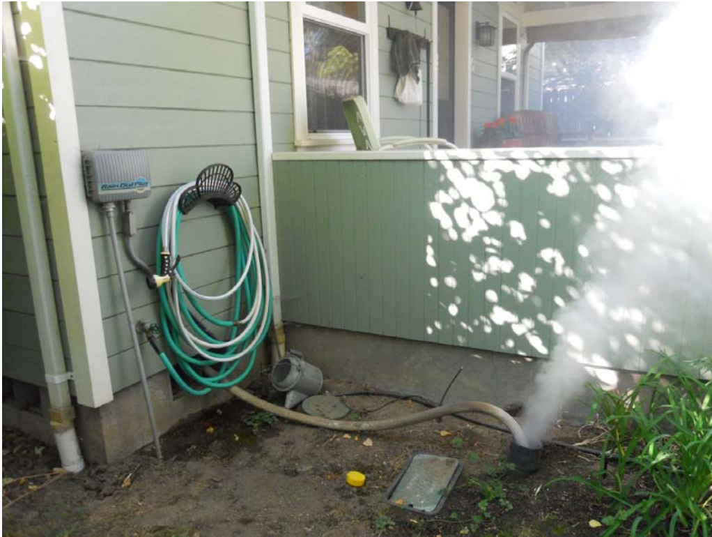
162 Harrison Street: Crawl space/basement sump pump discharging into sanitary sewer cleanout
