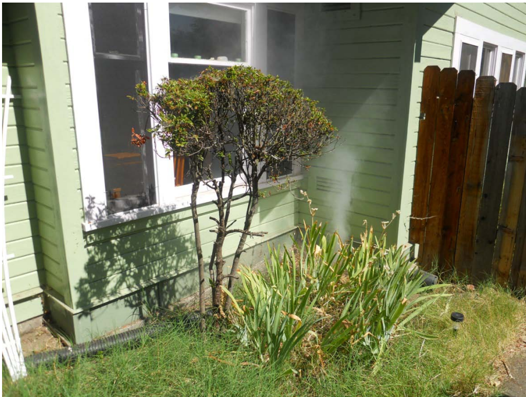
354 Liberty Street: Smoke emitting from cleanout with missing cap
