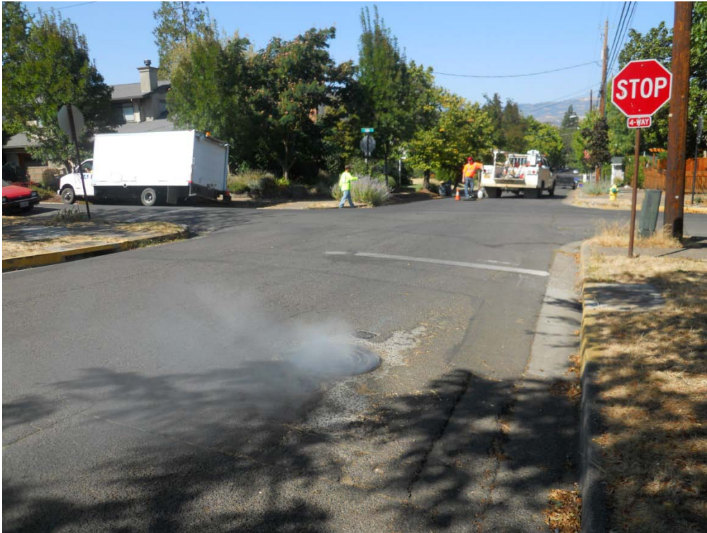
Smoke emitting from water PRV manhole located near Morton Street and Iowa Street Intersection
