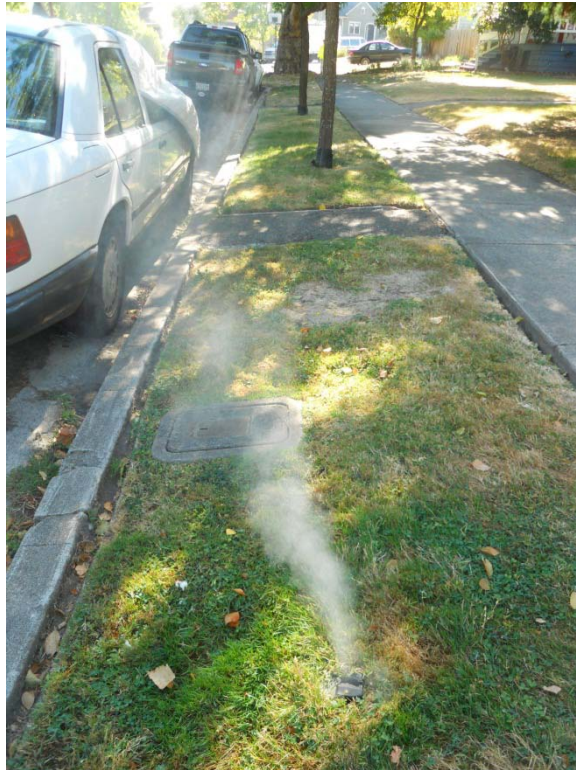
582 Allison Street: Smoke emitting from broken cleanout cap
