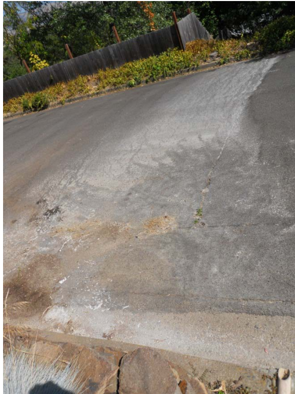
495 Jennifer Street: Laundry residue appears to be coming out of curb weep hole, clothes dryer could be connected to storm drain
