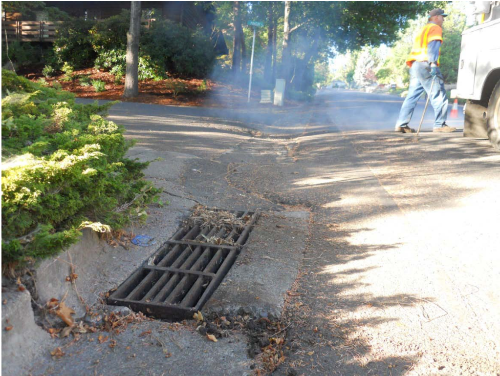
NE corner of Euclid Avenue and Pracht Street: Smoke emitting from catch basin
