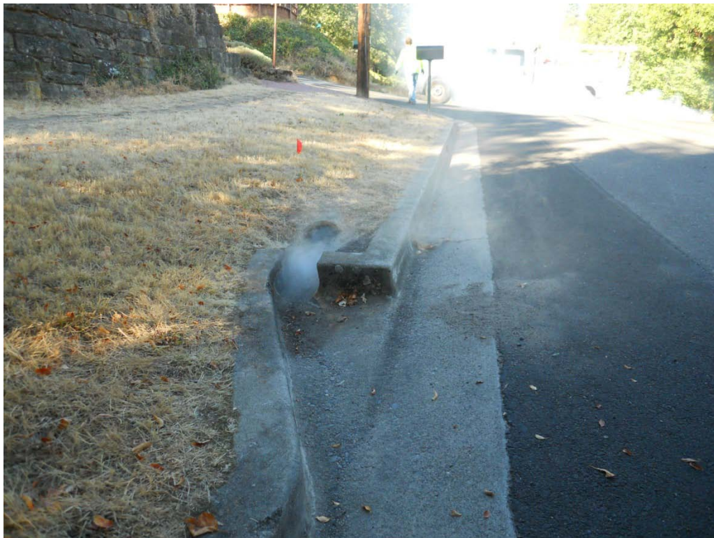
SE corner of Iowa Street and Gresham Street: Smoke emitting from abandoned storm pipe
