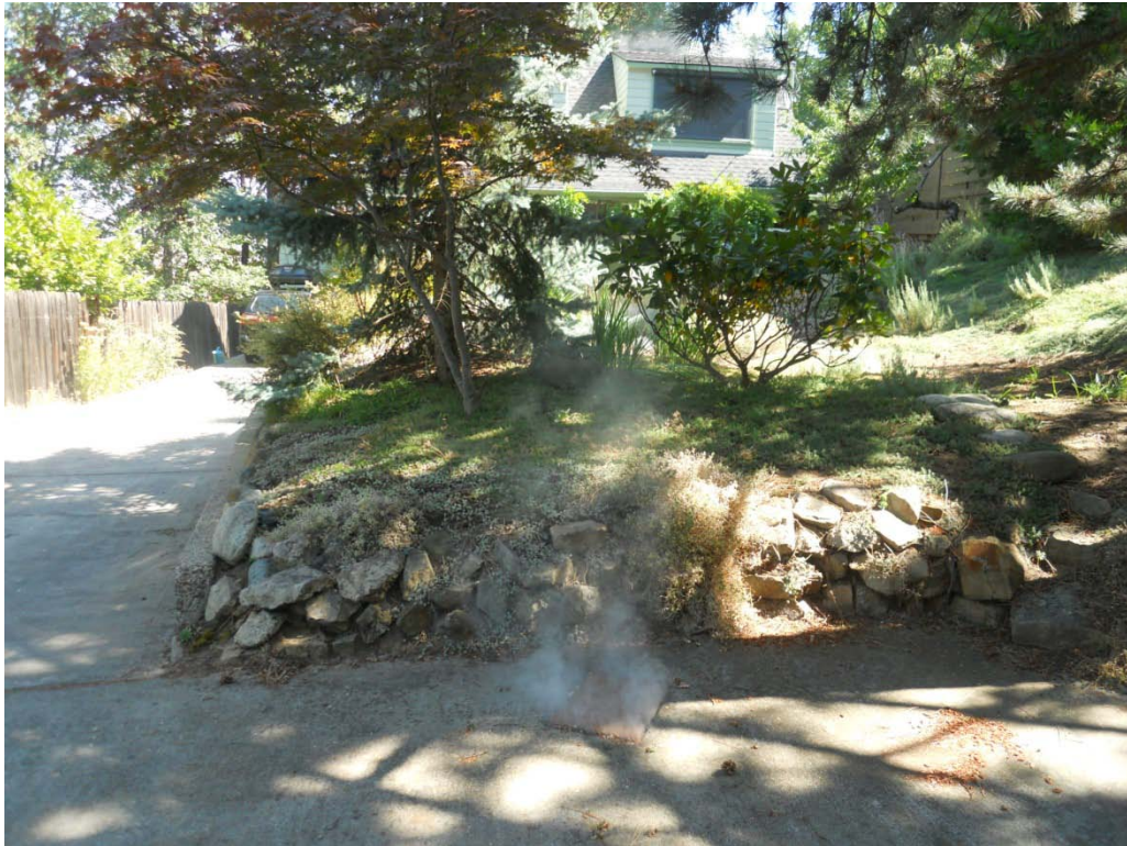
580 Mountain Avenue: Stone used in place of cleanout cap
