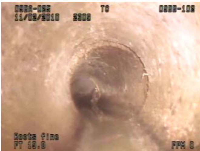
Pipe# 2309 Misaligned pipe
