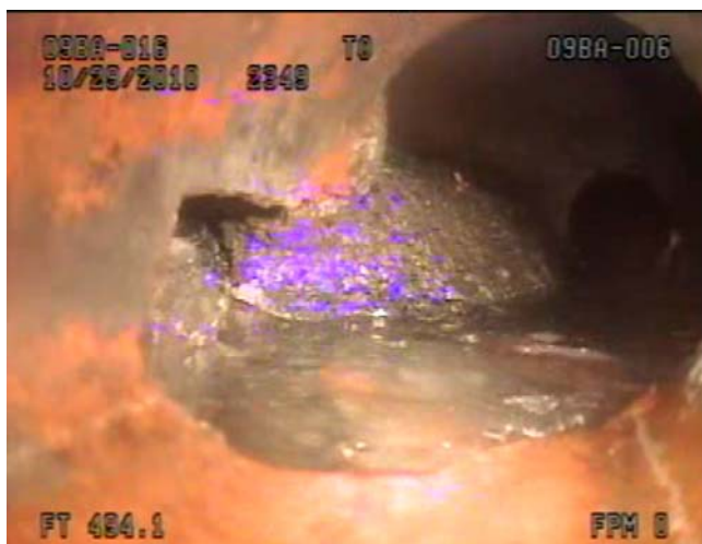
Pipe # 2349 Bottom of pipe missing
