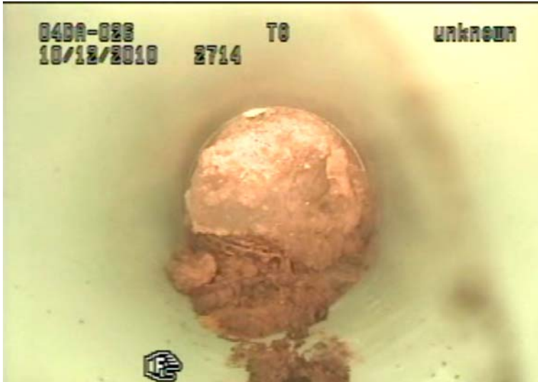
Pipe # 2714 -- Needs cap or manhole or clean out
