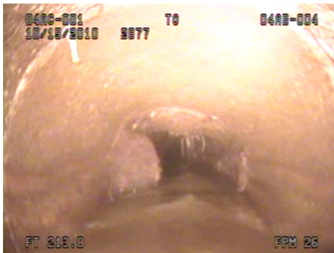
Pipe # 2877 Root mass; broken pipe
