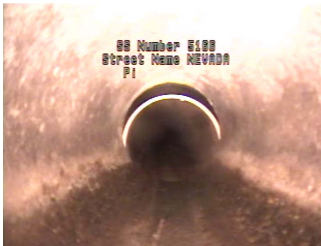
Pipe # 5166 Con/pvc transition; significant joint offset
