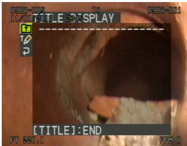
Pipe# 2345 Service crack and hole
