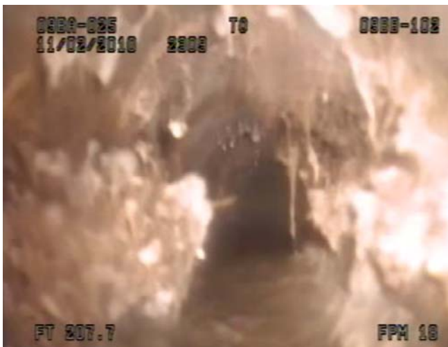
Pipe# 2309 Root mass; grease buildup
