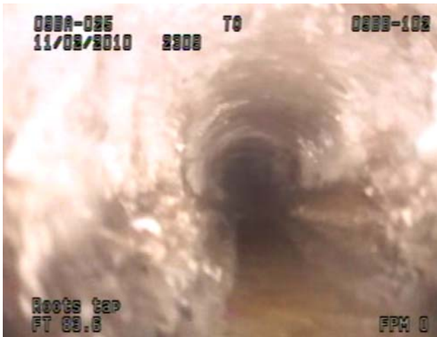
Pipe # 2309 Roots & grease buildup
