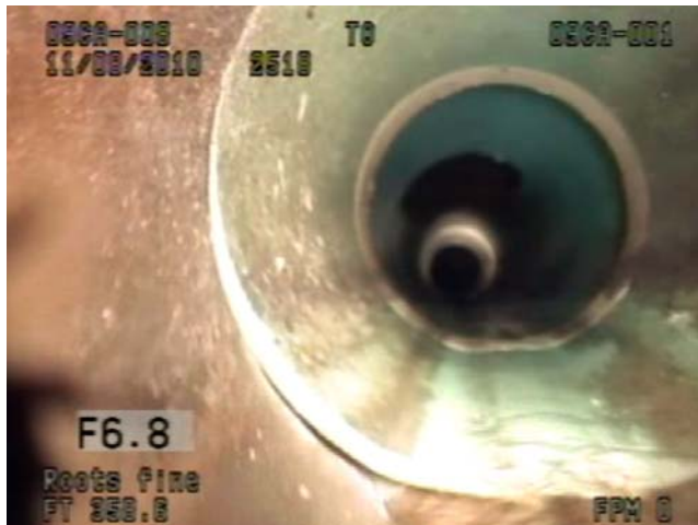
# 2518 Clay to pvc misaligned
