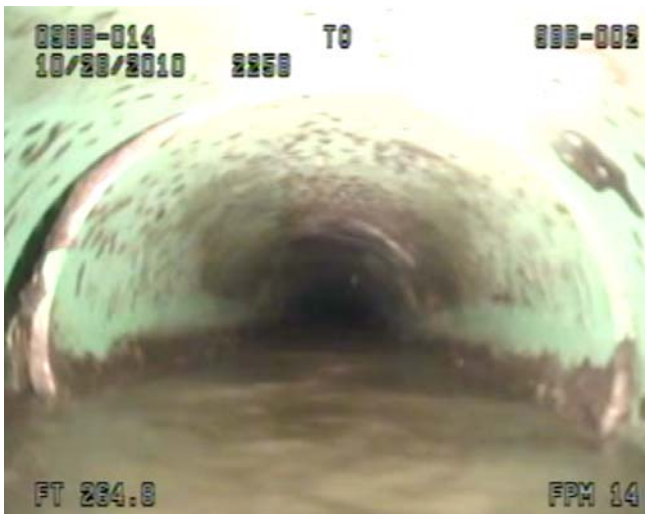
Pipe # 2258 Misaligned pipe
