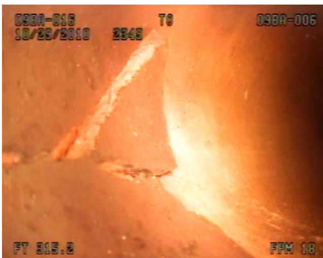
Pipe # 2349 Large crack at bell
