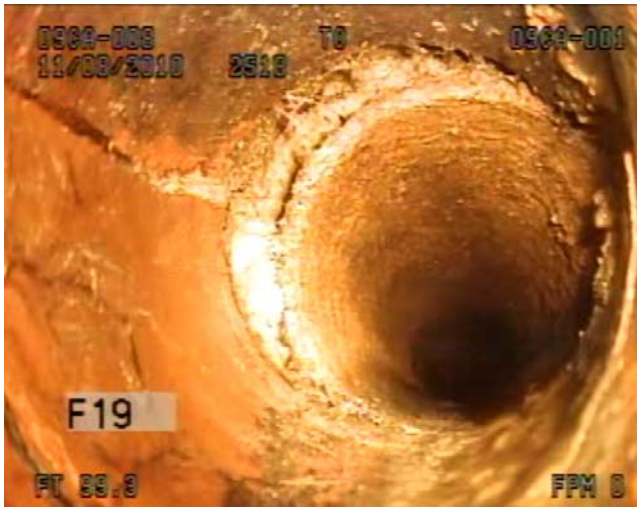
Pipe# 2518 Crack in service
