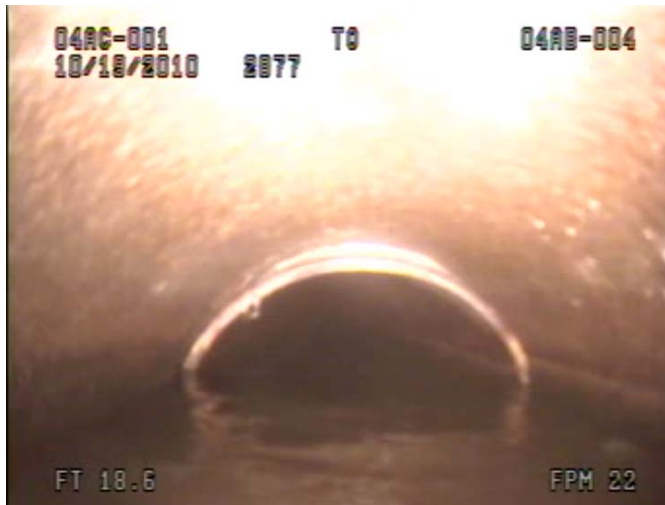
Pipe # 2877 Con/pvc transition; misaligned bell
