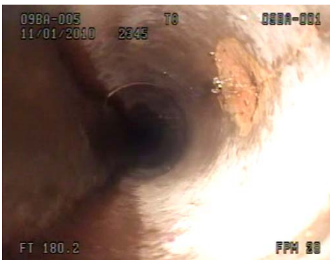
Pipe # 2345 Multiple cracks
