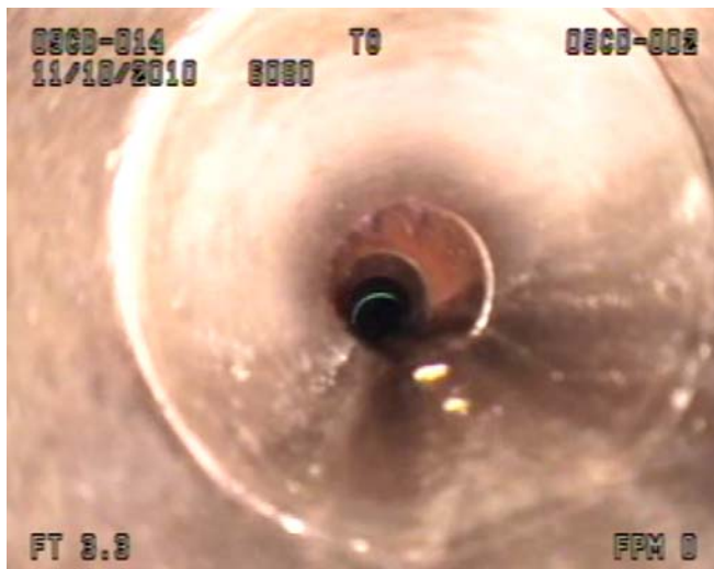
Pipe# 6080 Misaligned pipe
