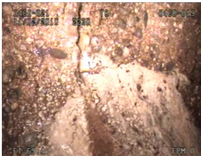
Pipe# 2230 Crack with infiltration
