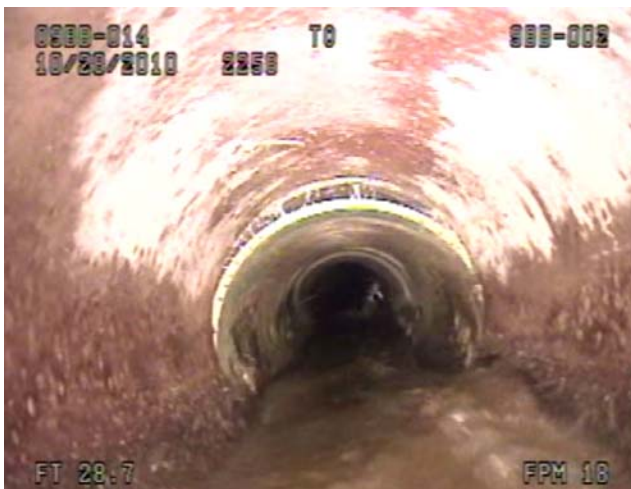
Pipe# 2258 Misaligned con/pvc
