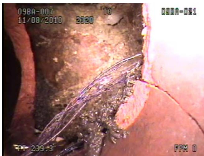
Pipe# 2328 Crack with missing pipe and roots
