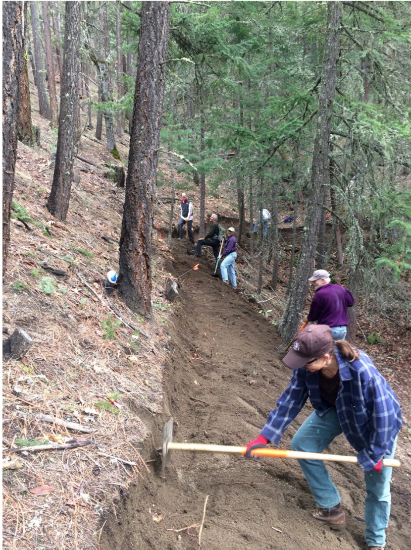
Figure 3-5: Trail work crew performing “rough-in” work on new Red Queen Trail.
