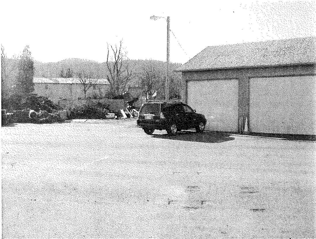
Photograph 1. Looking south toward the shop building and former location of underground storage tanks.
