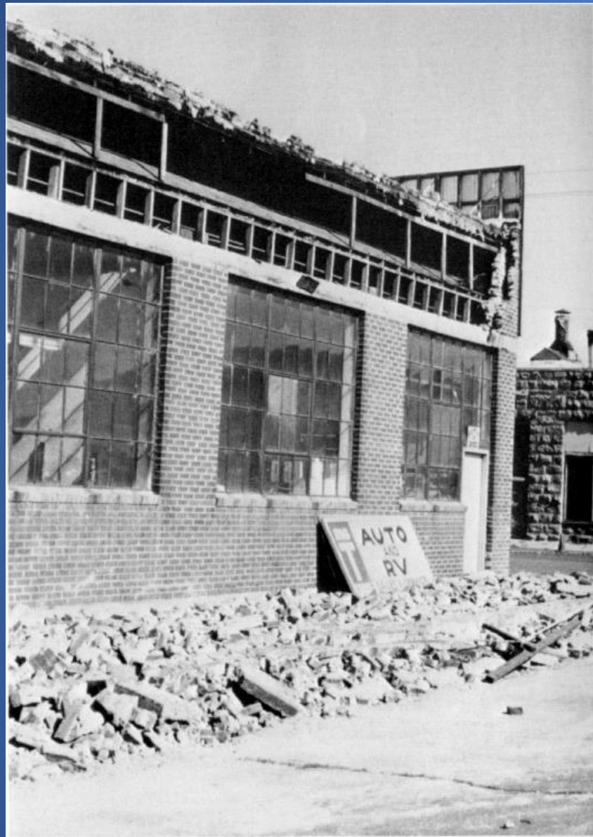
Klamath Falls, Oregon, earthquakes on September 20, 1993. Fallen debris litter the sidewalk beneath a partially collapsed, unreinforced-masonry wall and parapet in downtown Klamath Falls.
