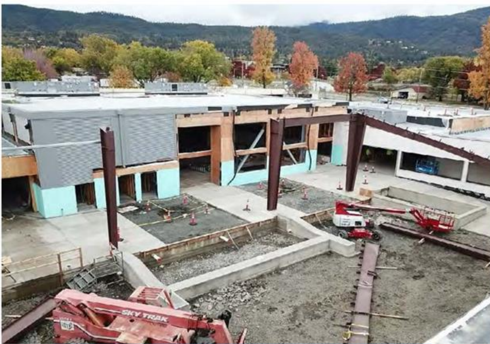
COURTYARD/CANOPY PROGRESS AT ASHLAND MIDDLE SCHOOL
