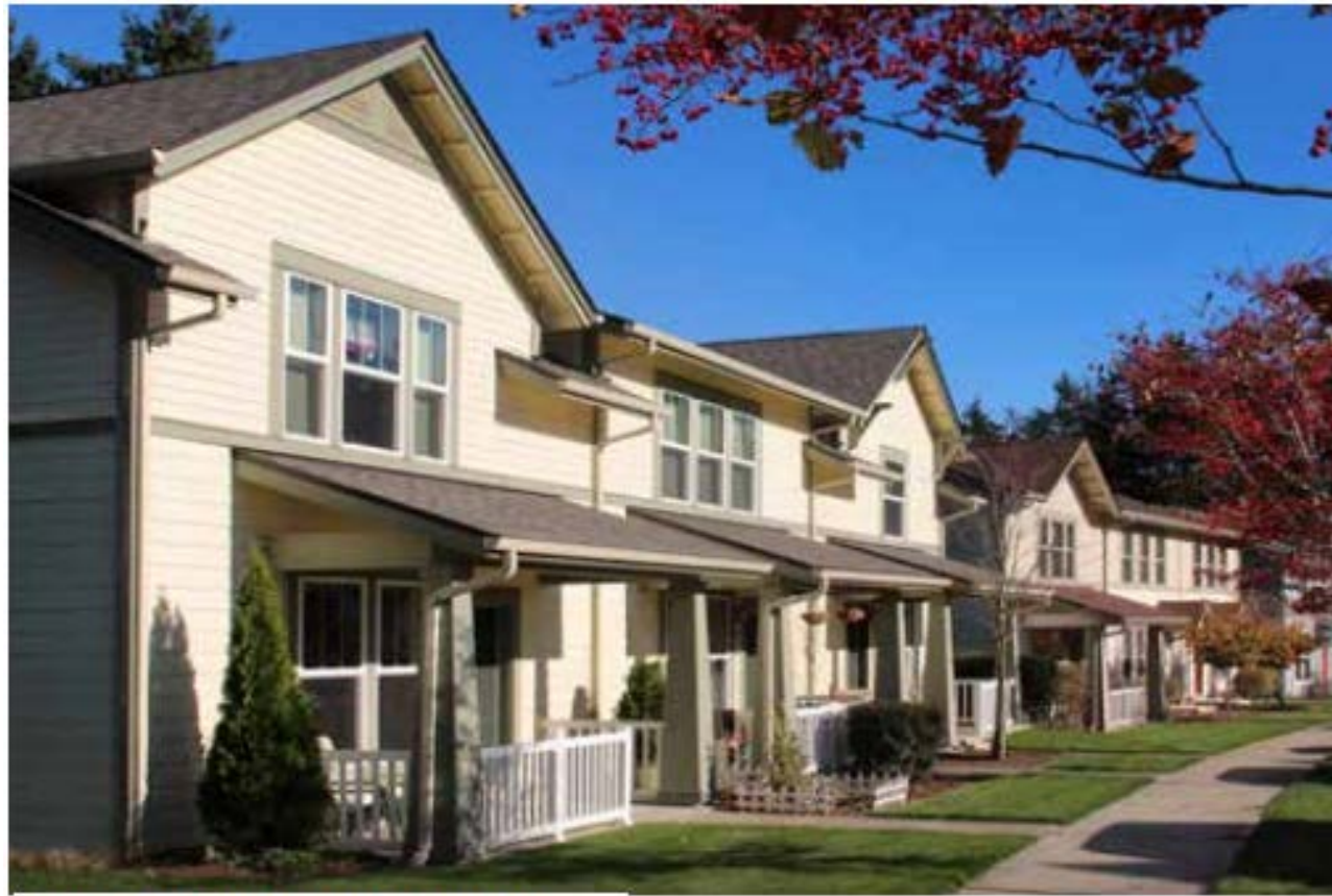
Side-by-side duplex, Tacoma, WA Torti Gallas + Partners
