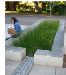
STORM WATER FEATURE
