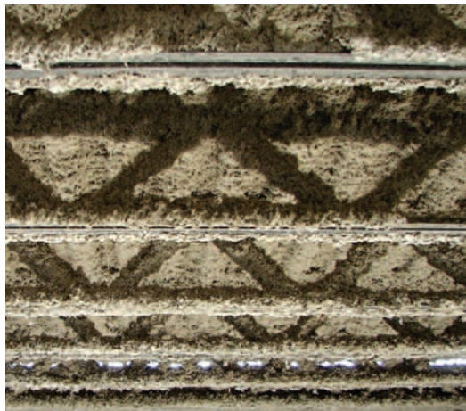
Figure C-4: Fireproofing added to structural steel
