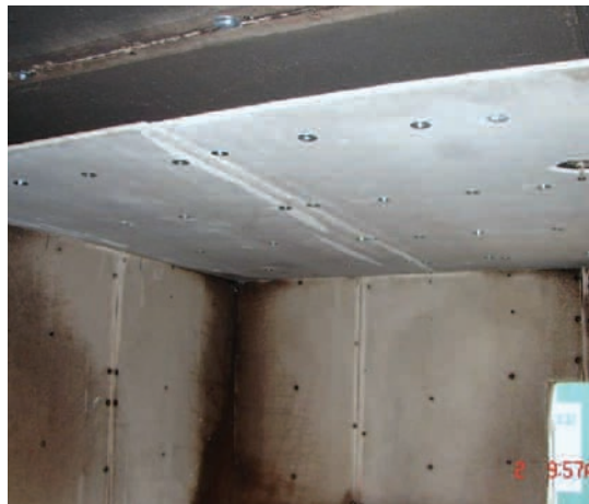
Figure C-5: Additional construction of burn room walls and ceiling and deluge sprinkler head.
