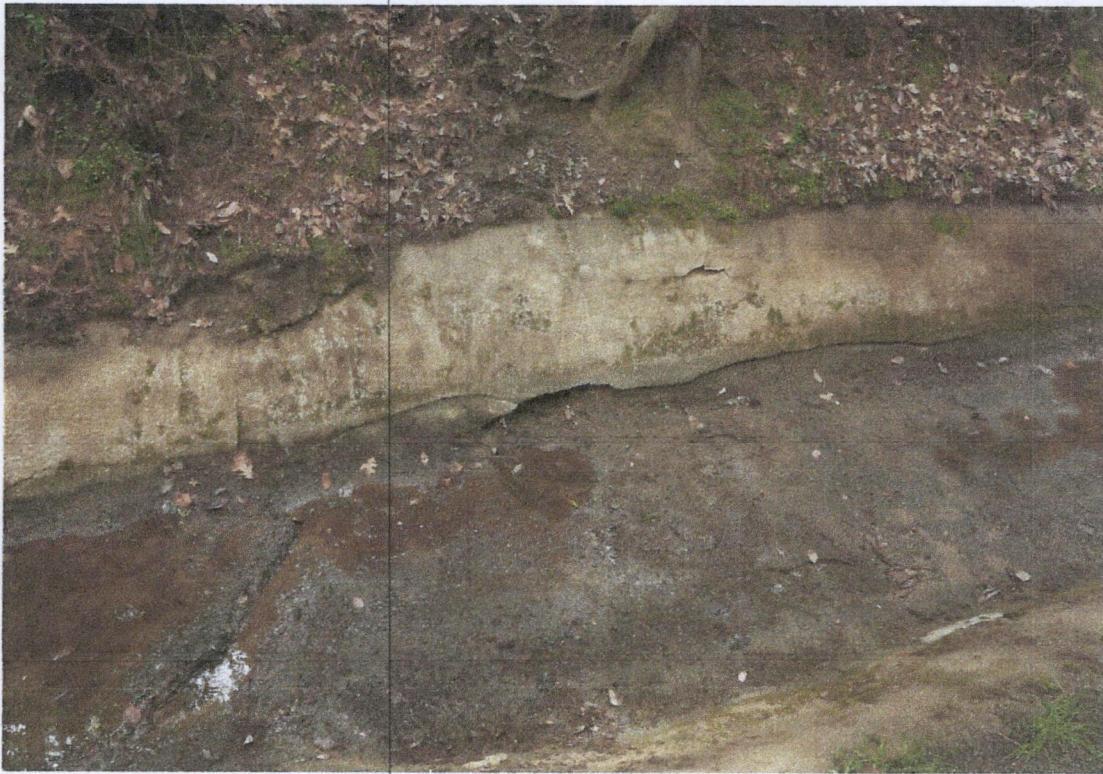
4-7-2019 Close-Up of canal after city and county crews have done the spring cleaning
