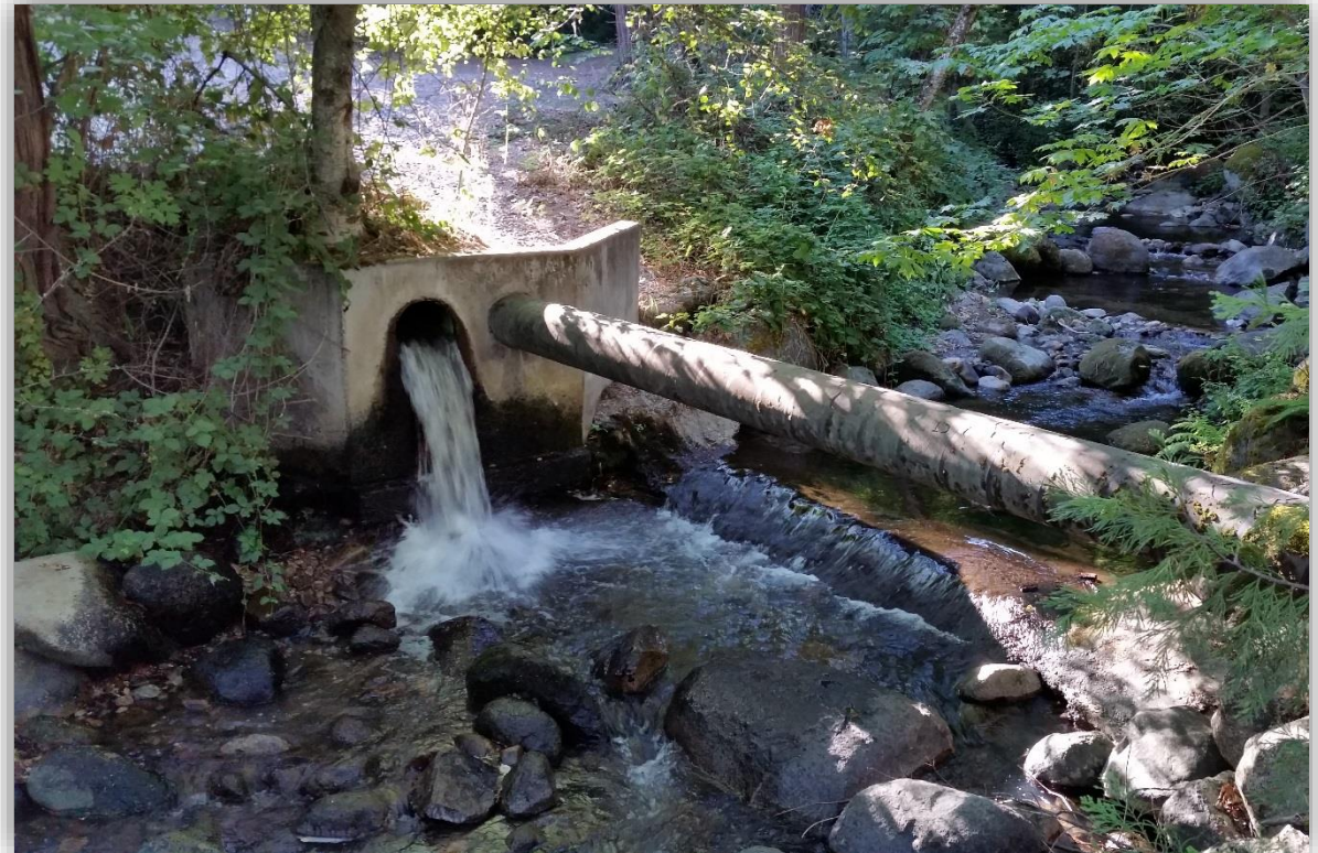
Ashland Creek – Ashland Canal Outfall
