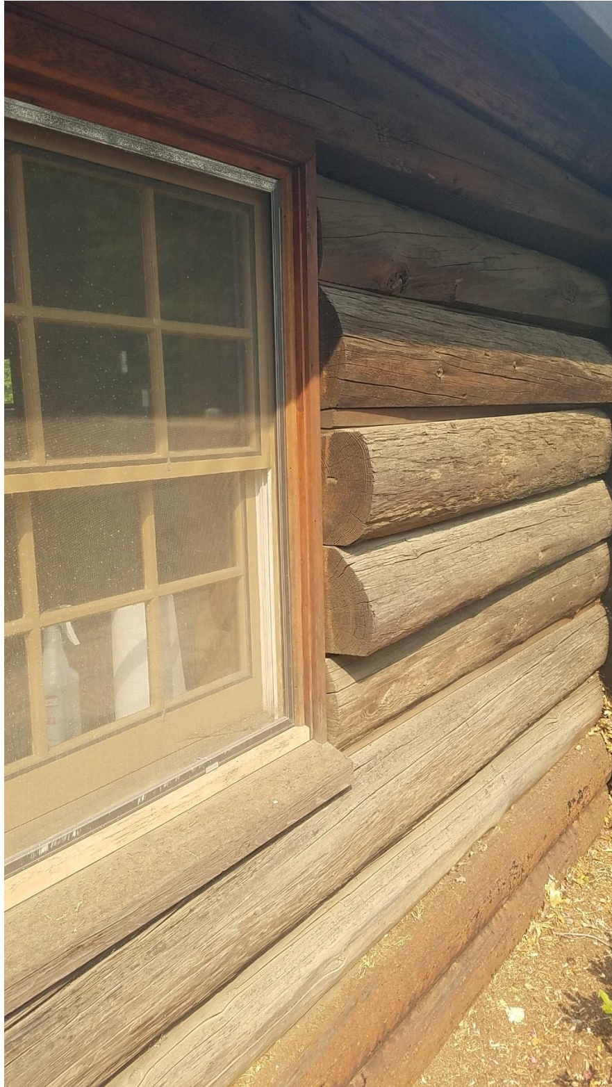
Figure 9. Pioneer Log Cabin, "Unpinned" Logs at SE Corner Window
