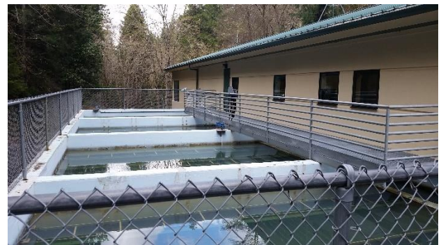
Ashland Creek WTP
