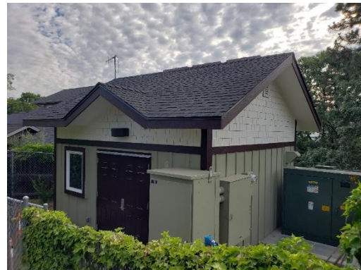
Terrace Street Pump Station
