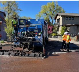
selected for slurry seal treatment are commonly those which have slight to moderate distress, no rutting, and generally narrow crack widths, and where a slurry seal treatment would help extend the pavement life until resurfacing becomes necessary.
